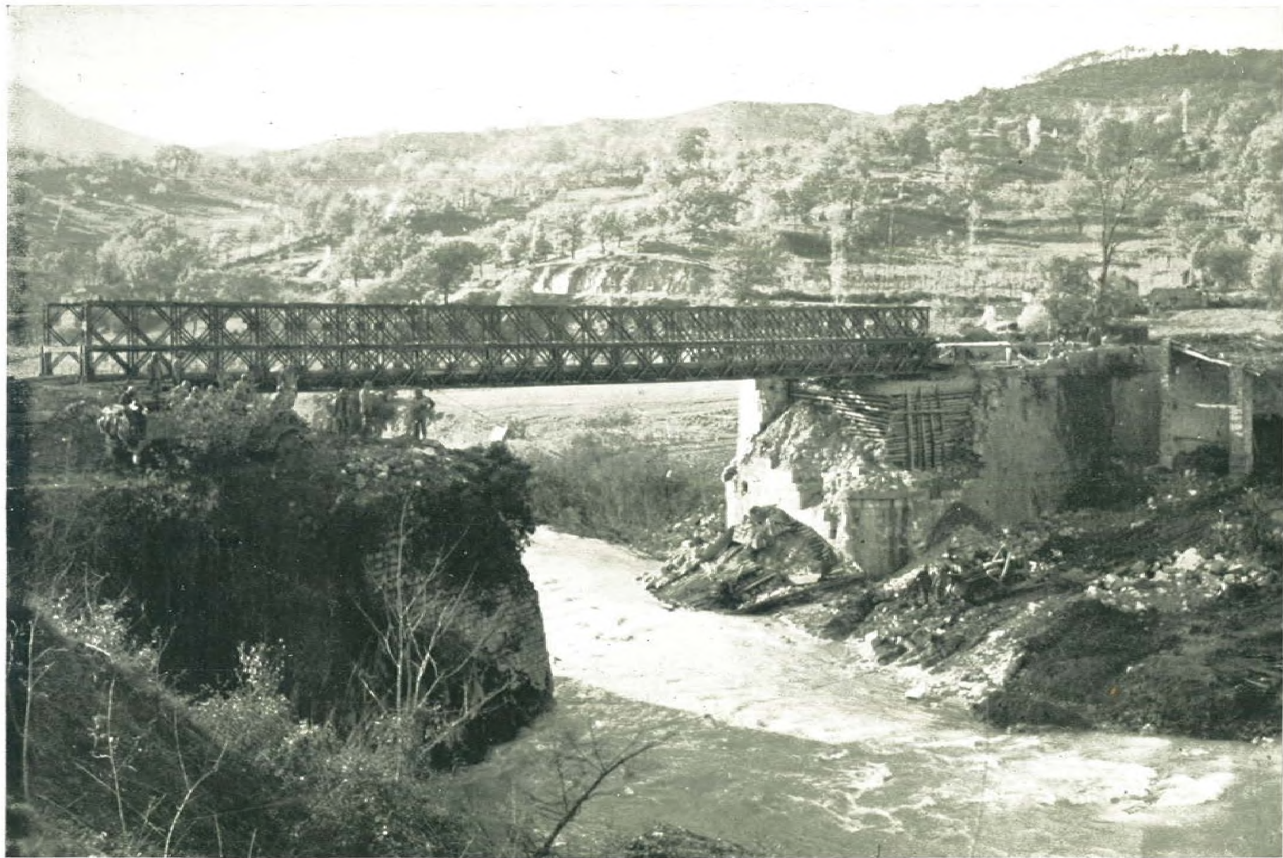
The Ritter Bridge at Colli
