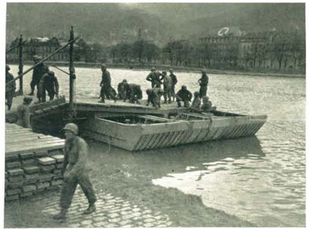
"Near Shore Transom In Place"
