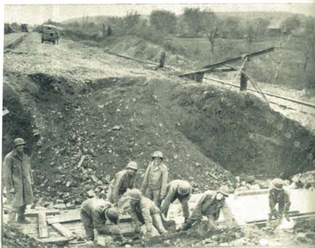
Culvert On Highway 48
