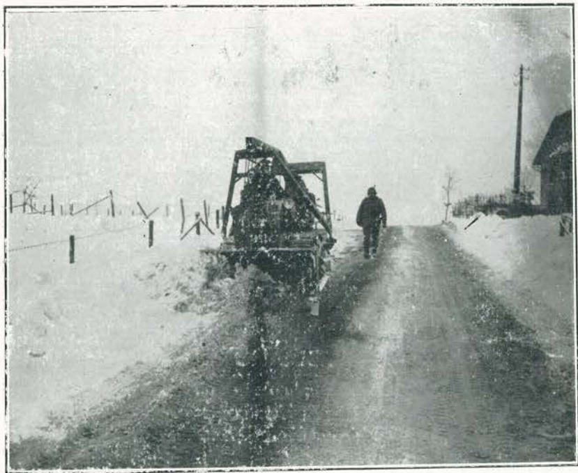
CLEARING SNOW FROM ROADS, ST. VITH
