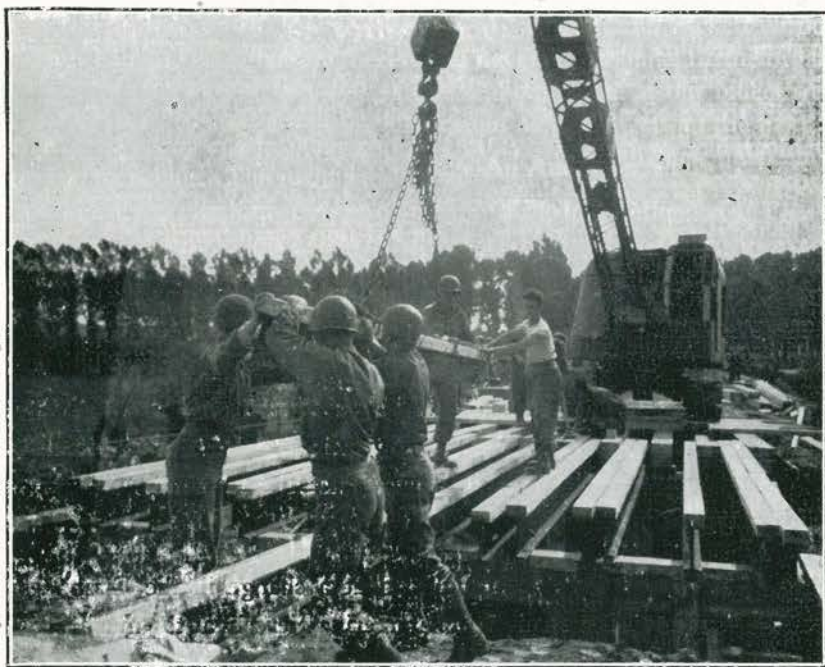
CONSTRUCTION OF STANDARD BRIDGE AT MOXHE, BELGIUM
