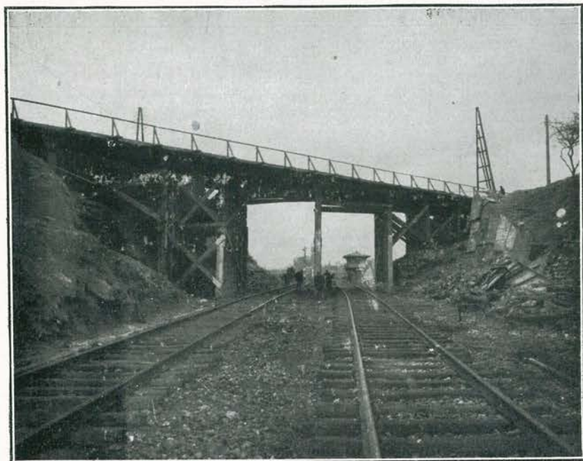
TRESTLE BENT BRIDGE, ARLON
