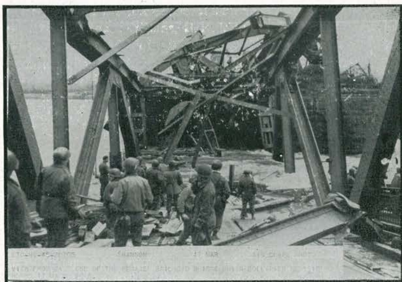
REMA GEN BRIDGE SHORTLY AFTER COLLAPSE
