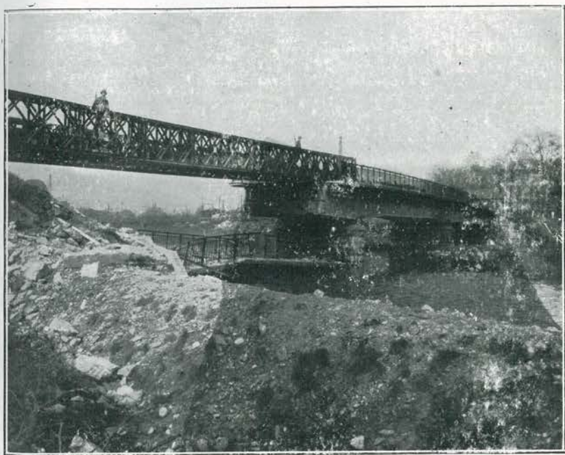
BAILEY BRIDGE AT OVENTROP, GERMANY
