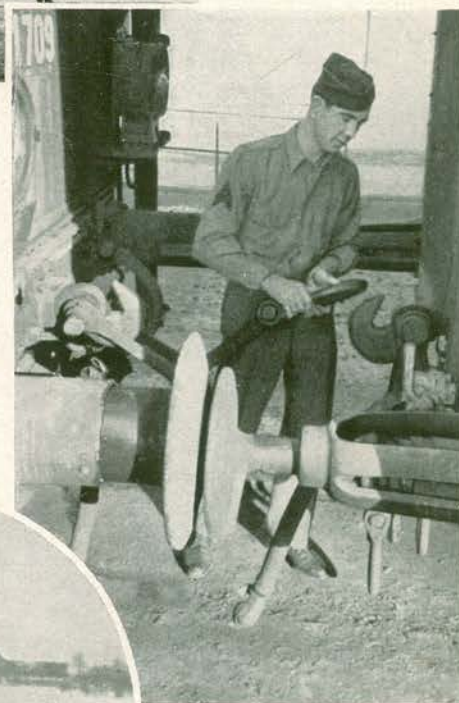
Right: Link and pin coupling—Sgt. McHale
