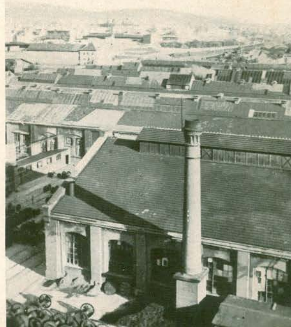
Corner: Locomotive back shop, Esslingen
