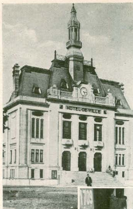
Above: City Hall, Aulnoye
