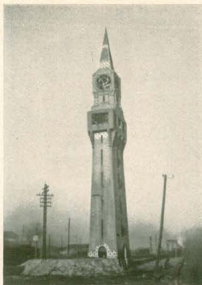
Above: Tower, Aulnoye
