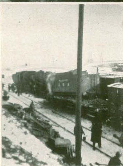
Left: Caboose telescoped by tender, Aulnoye
