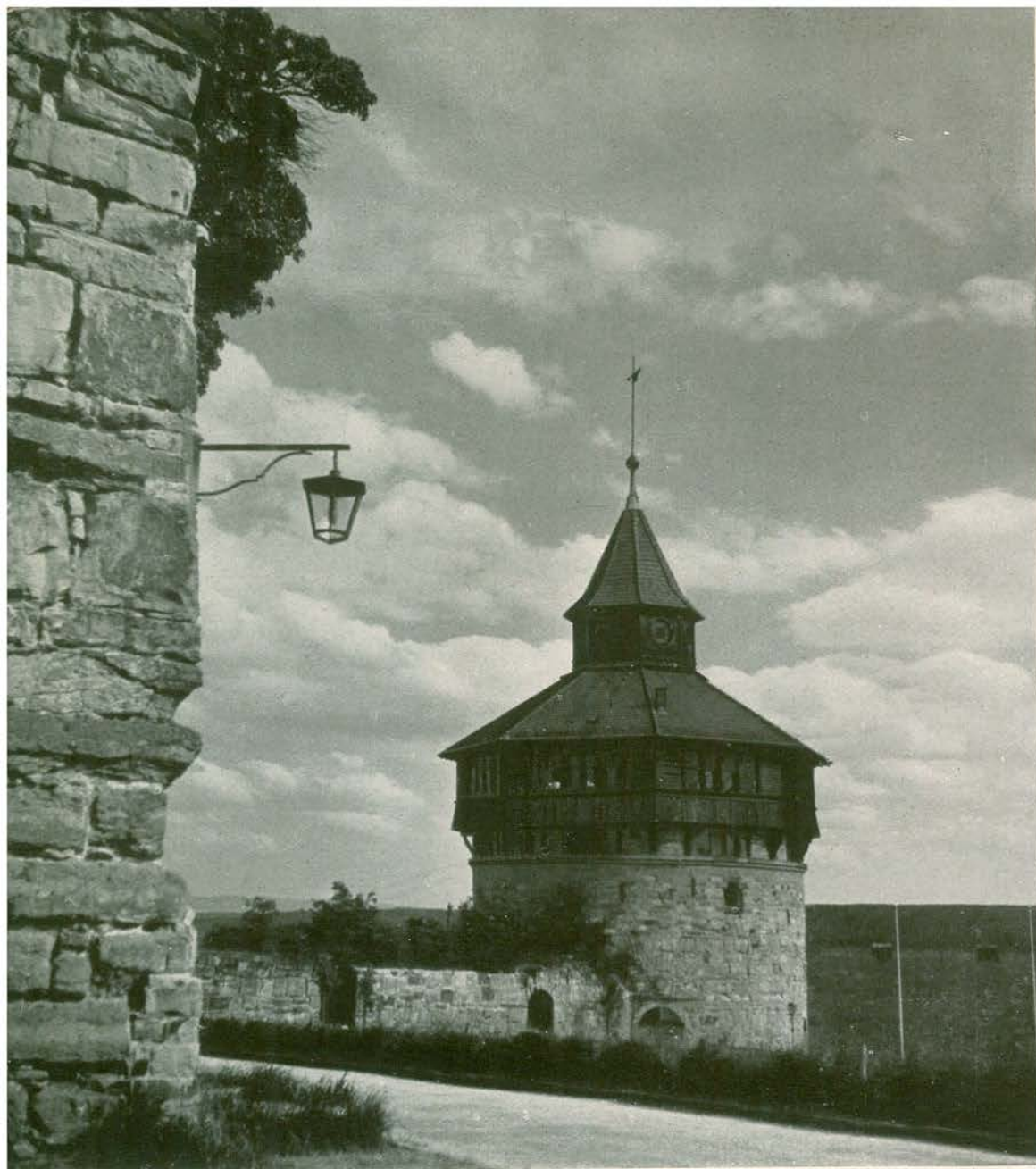
Above: Tower, Esslingen
