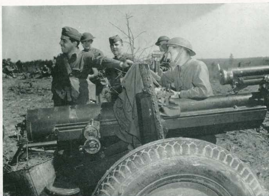
Left: Shifting the trail. Below: The base deflection is checked on a 37-mm. gun.
