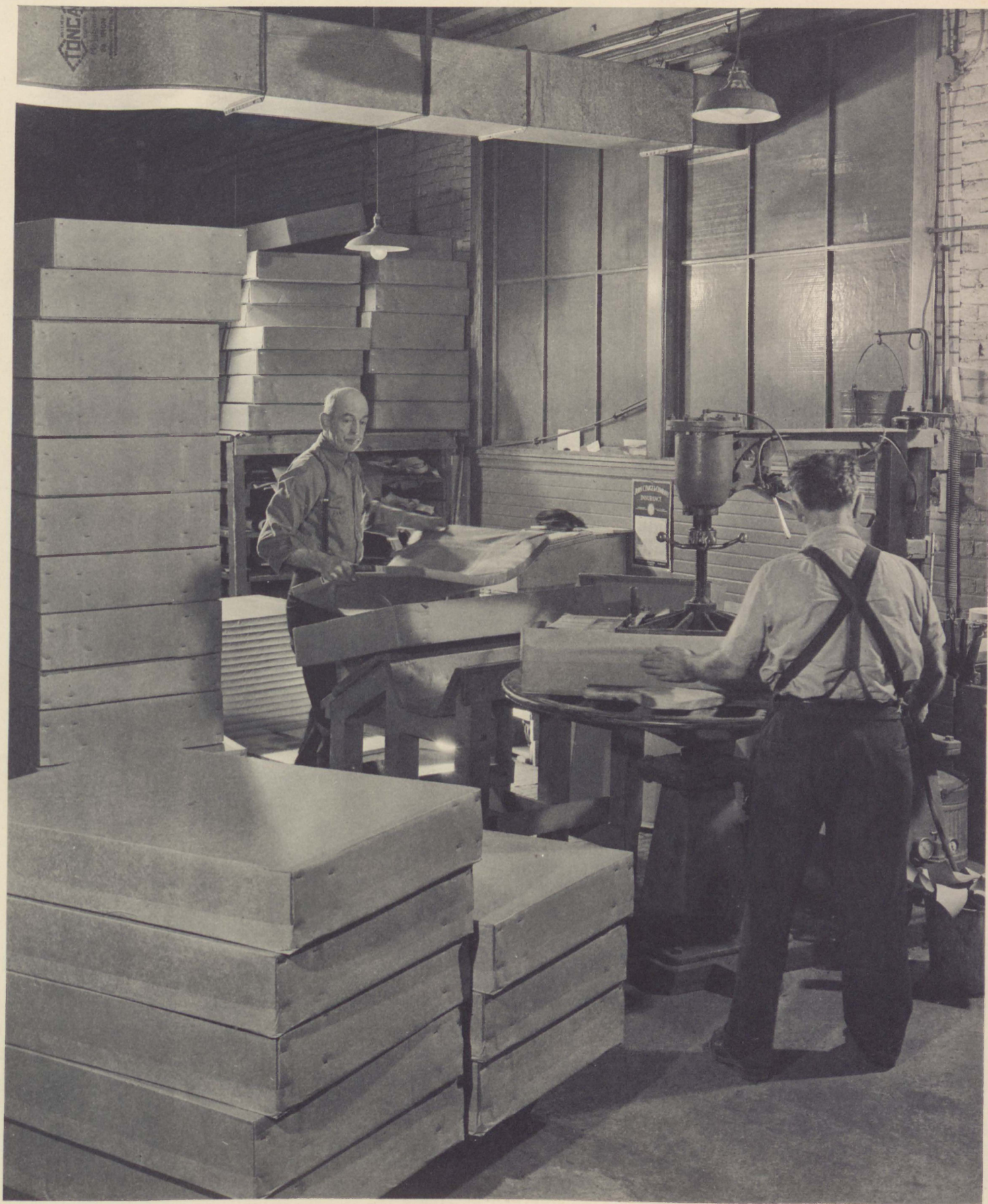
The finishing touch is added by George Fish and Leo Emerson who package reams with an hydraulic packing machine . . . a modern device that forces air out of cartons, and assures a strong sealed package.
