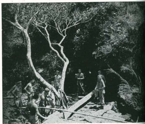
The damned dam broke last night.
