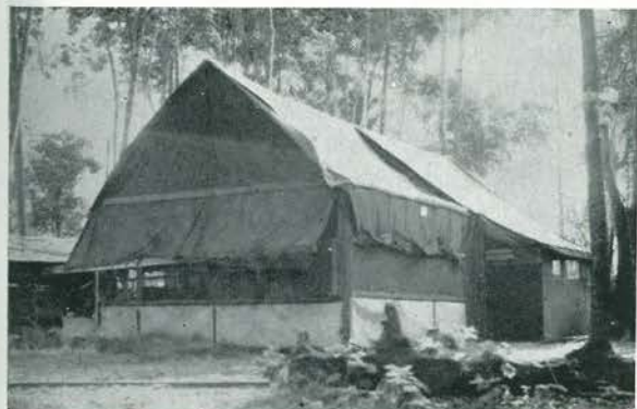
Operations and Intelligence Building.
