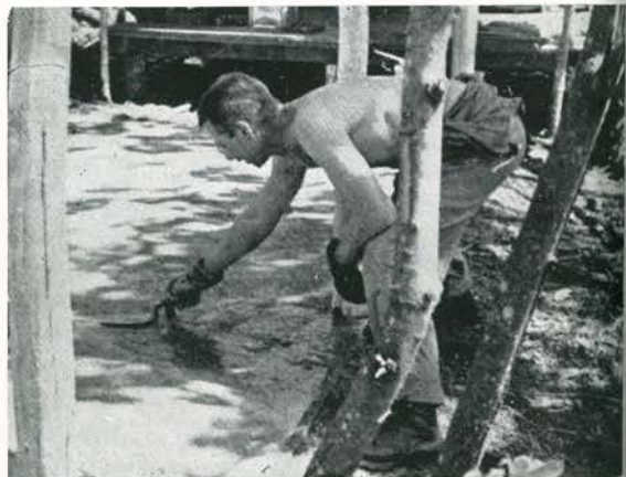
On this spot will stand the Dispensary.
