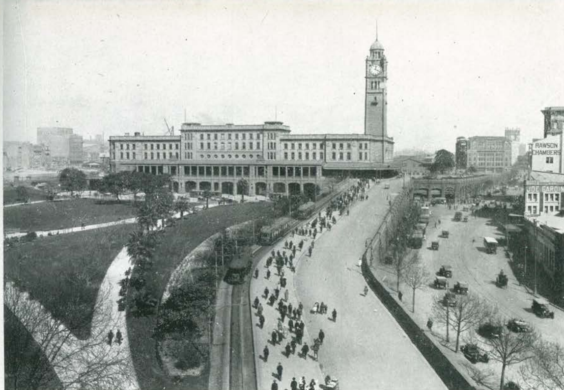
Central Railway Station, Sydney.
