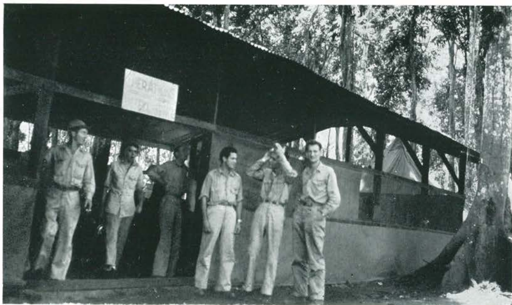
Operations and Intelligence building.
