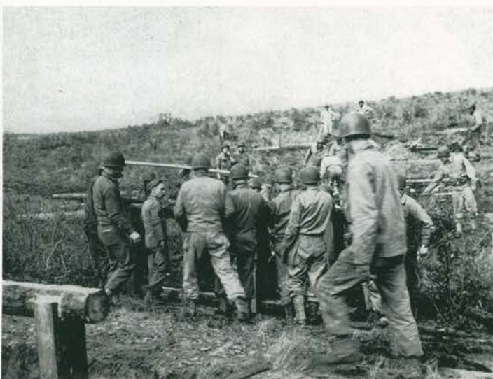
As Bridge progresses, Sgt. Gainer explains the construction and centering of one bent
