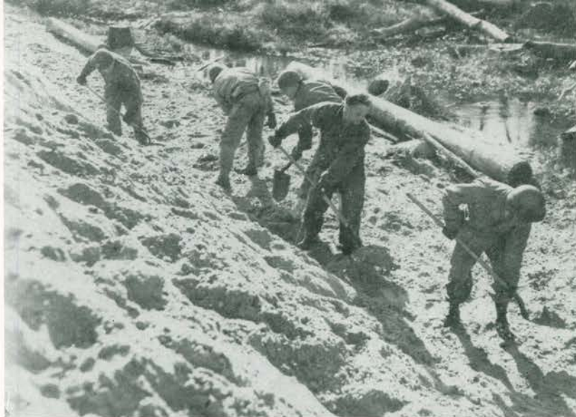
Company A—Constructing the approach to an expedient Ponton Bridge, to cross Drowning Creek
