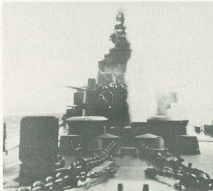
GEYSER COMING FROM HATCH ON FO'S'LE, OPENED TO RELIEVE PRESSURE CAUSED BY TORPEDO HOLE IN BOW
