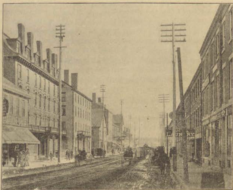
EXCHANGE STREET, LOOKING TOWARD RIVER.
