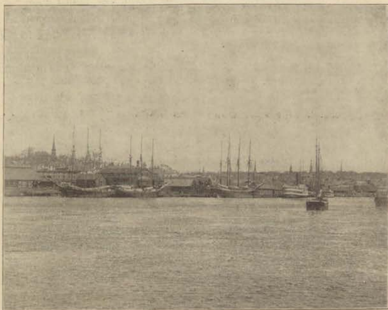
BANGOR WATER FRONT, BELOW BRIDGE.
