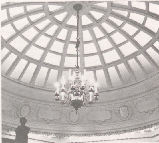
Interior Dome and Chandelier
