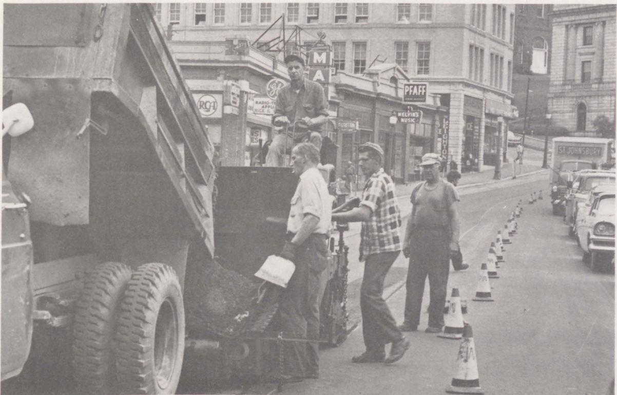
Paving Machine in Action
