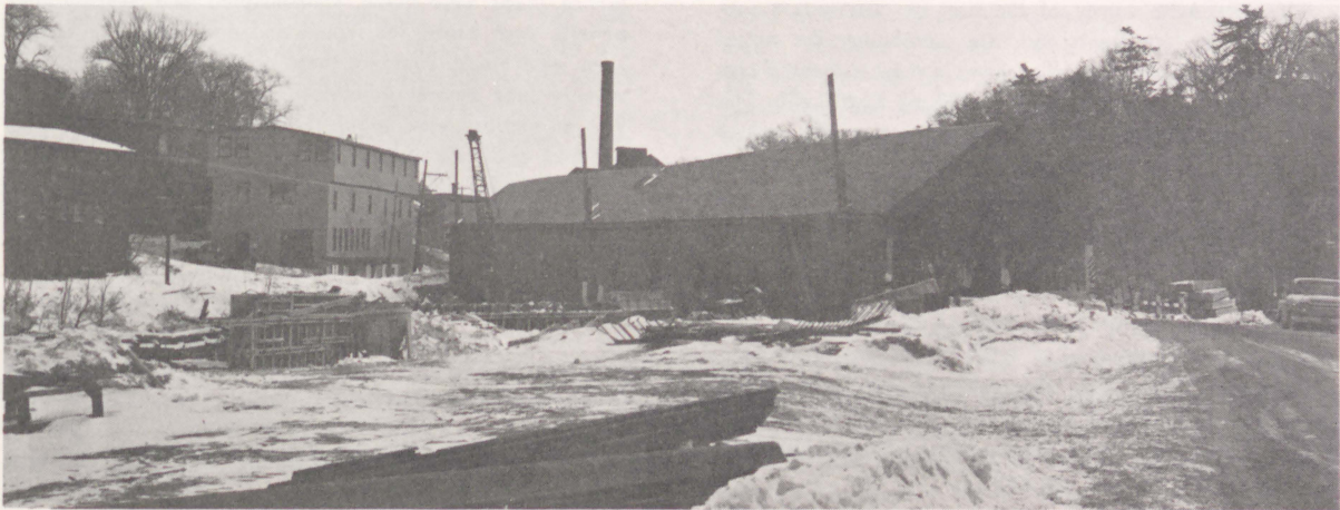
The Reconstruction of Moses Bridge Begins
