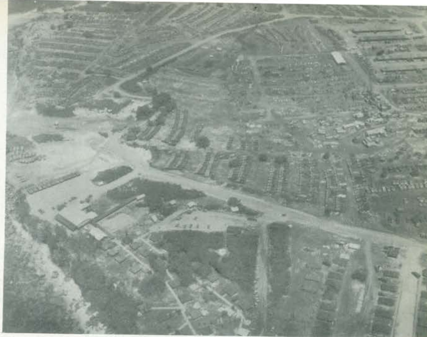
Aerial view, Base M.
