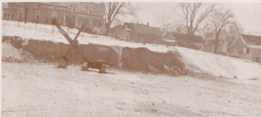
Newbury Street Playground under Construction
