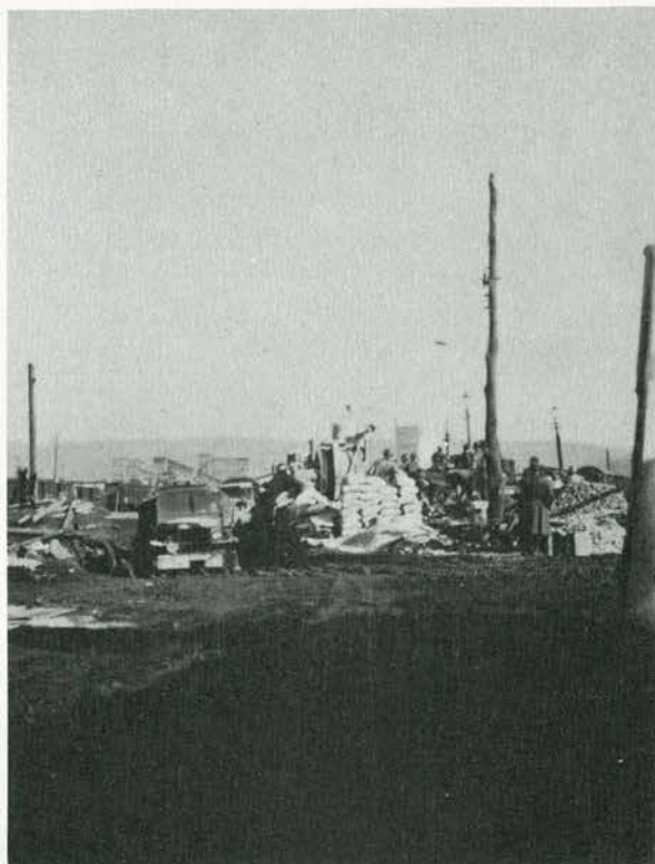
Remember Lt. Merrick's concrete mixing plant?
