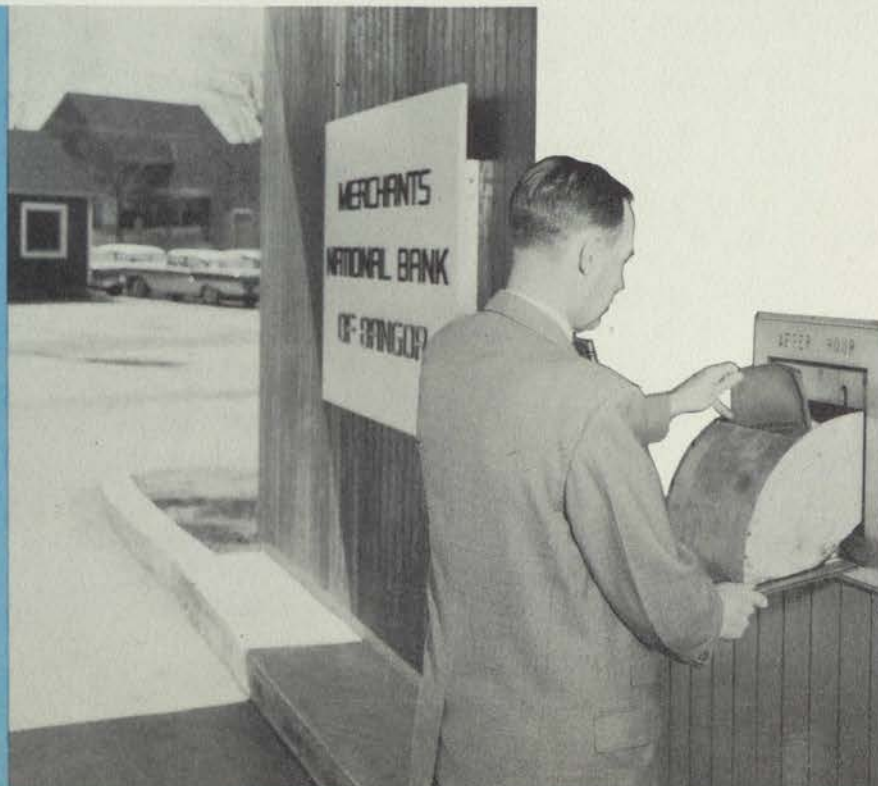
Union Street Office
