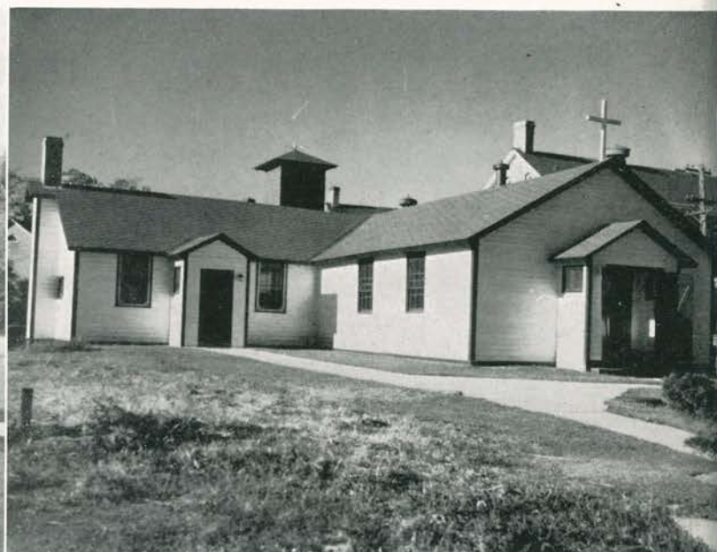
Post Chapel, Fort McKinley.
