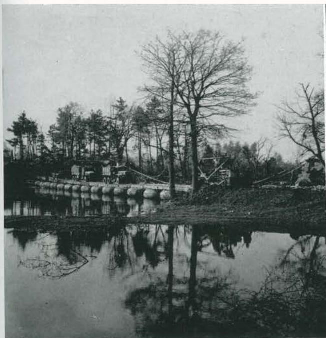
228-foot floating treadway over Aggar at Seigburg
