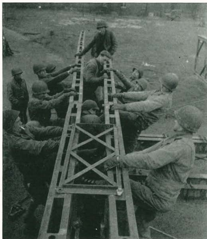
Double Double Bailey bridge being launched by Company A at Wanssum, Holland
