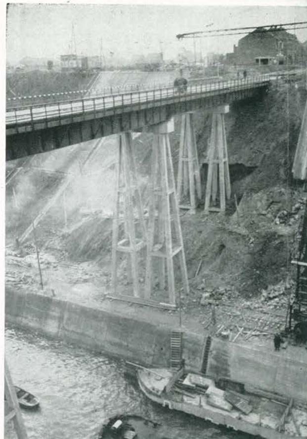
The Albert Canal near Maastricht, Holland, shows where temporary bridge has been placed beside dropped permanent bridge on background. This is a few miles north of Eben Canal
