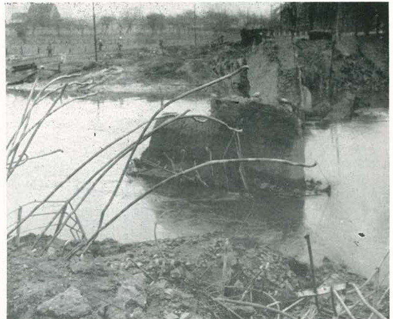
Bridge demolished across the Lippe River
