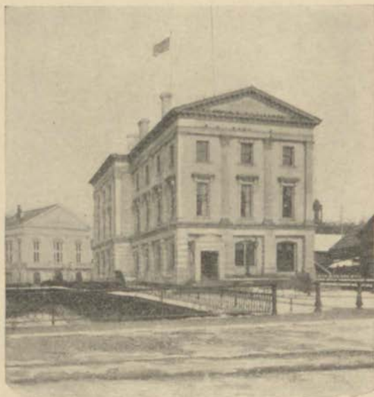
CUSTOM HOUSE AND POST OFFICE.
