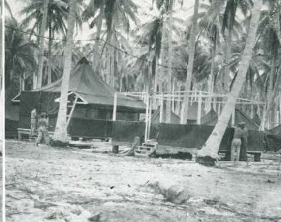
Tents under construction. Coconut logs cut in our own sawmill furnished lumber for framing.
