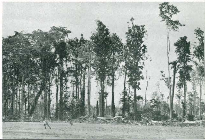
Bulldozers aided in clearing this baseball diamond. The Group nine was good enough to take the Sansapor Series.
