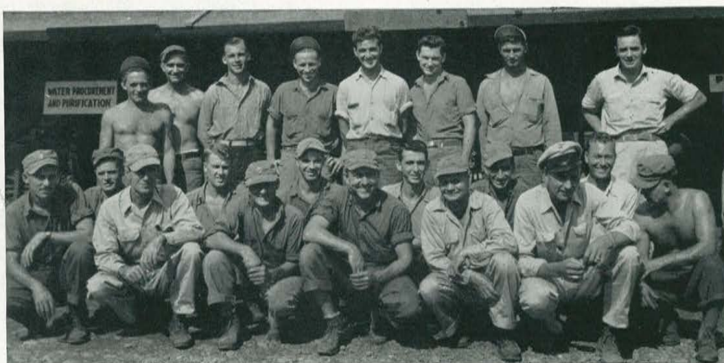
Water Department Crew
