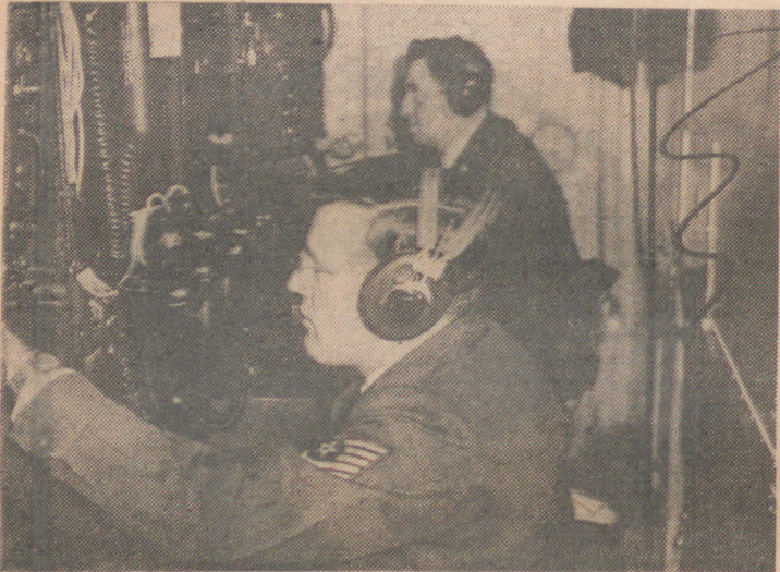
INITIAL CONTACT —Initial contact with incoming aircraft is made by men in the GCA Unit. The final controller, using precision radar vectors the aircraft and issues altitude and heading corrections.
