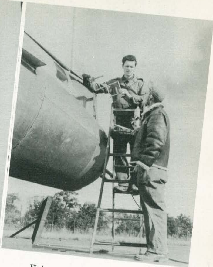
Fixing a flak hole — Station 131
