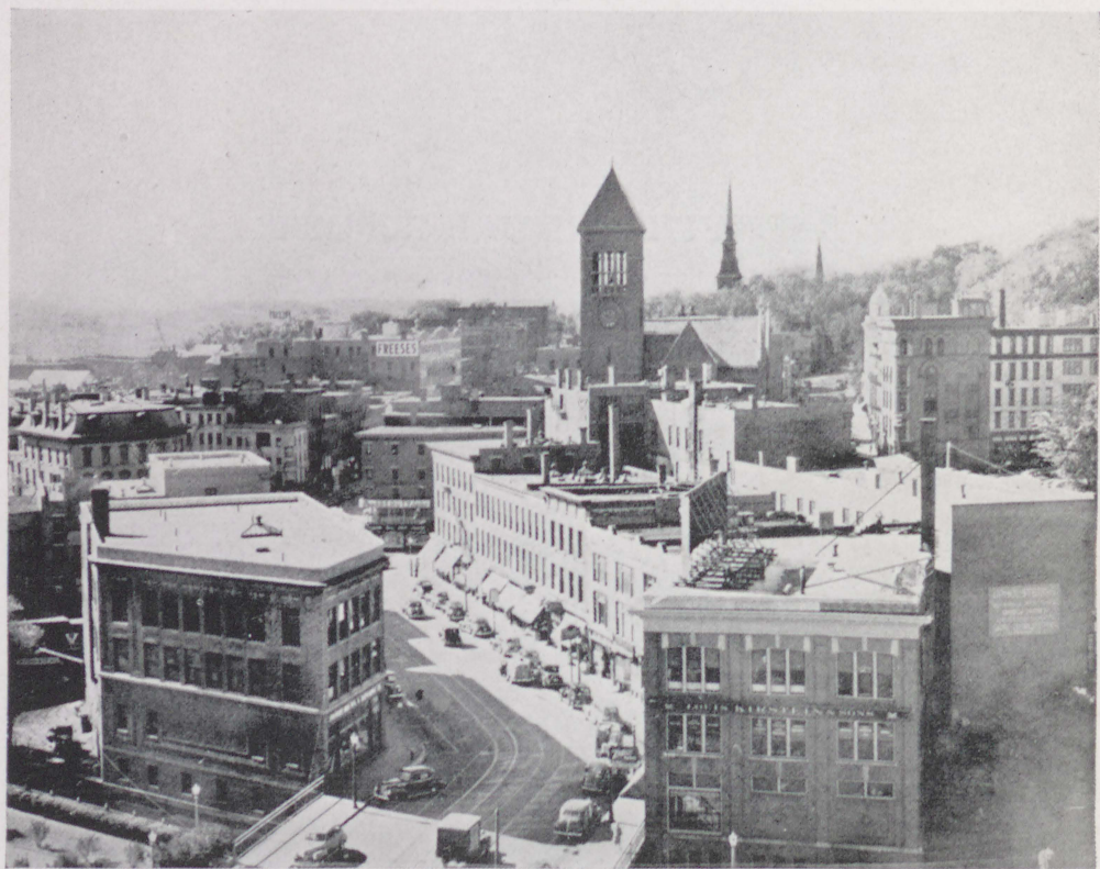
PARTIAL VIEW OF CITY OF BANGOR LOOKING SOUTH ON CENTRAL STREET
