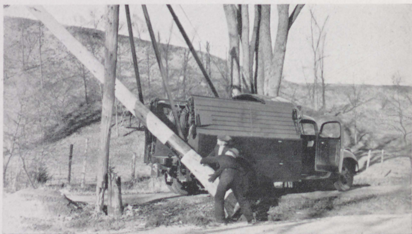
LINE CREW OF ELECTRICAL DEPARTMENT REPLACING BROKEN POLE
