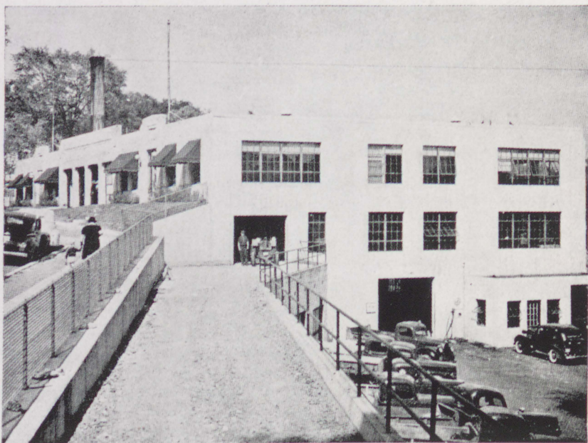
PARTIAL VIEW OF MUNICIPAL GARAGE
