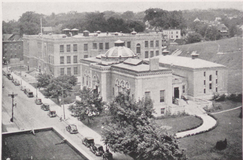
VIEW OF BANGOR PUBLIC LIBRARY WITH BANGOR HIGH SCHOOL IN THE BACKGROUND
