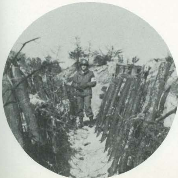
Trench—Frankfurt Race Track
