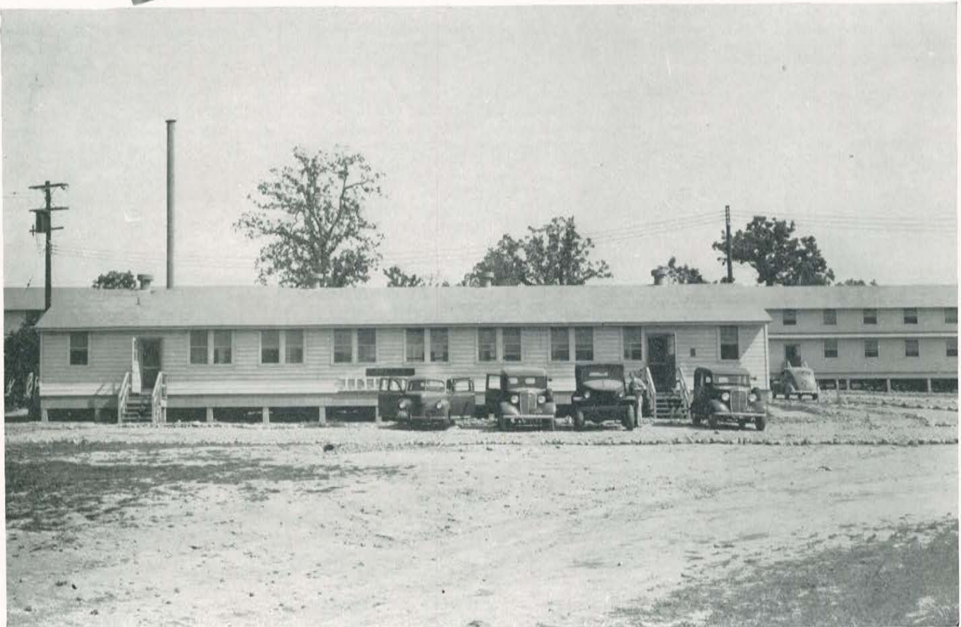
Regimental Headquarters Building.
