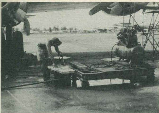
After this first mission, maintenance continued, . . .
