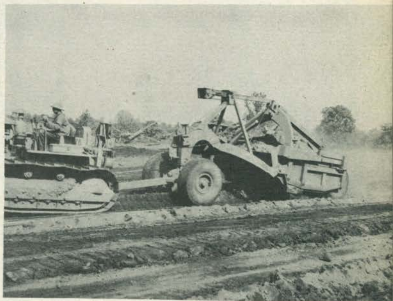
while construction work . . .
