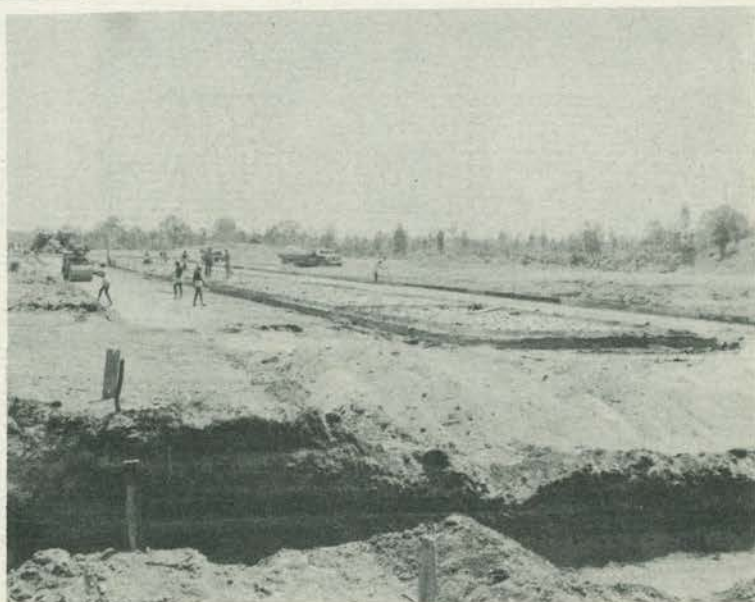
building the new taxiway . . .
