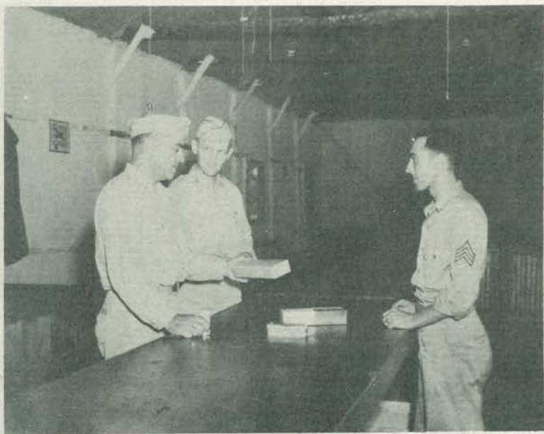
inspected the base.
