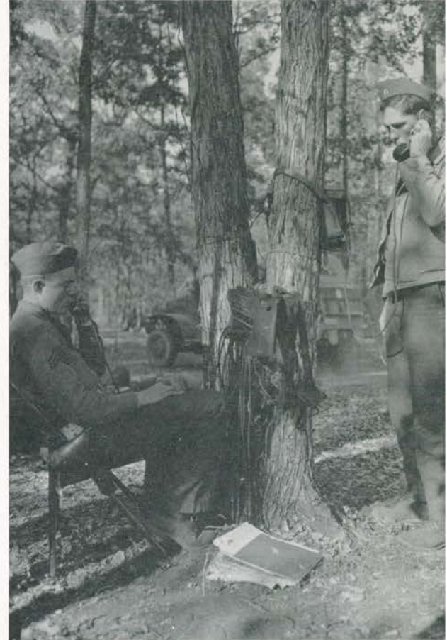
Switchboard in the field.
