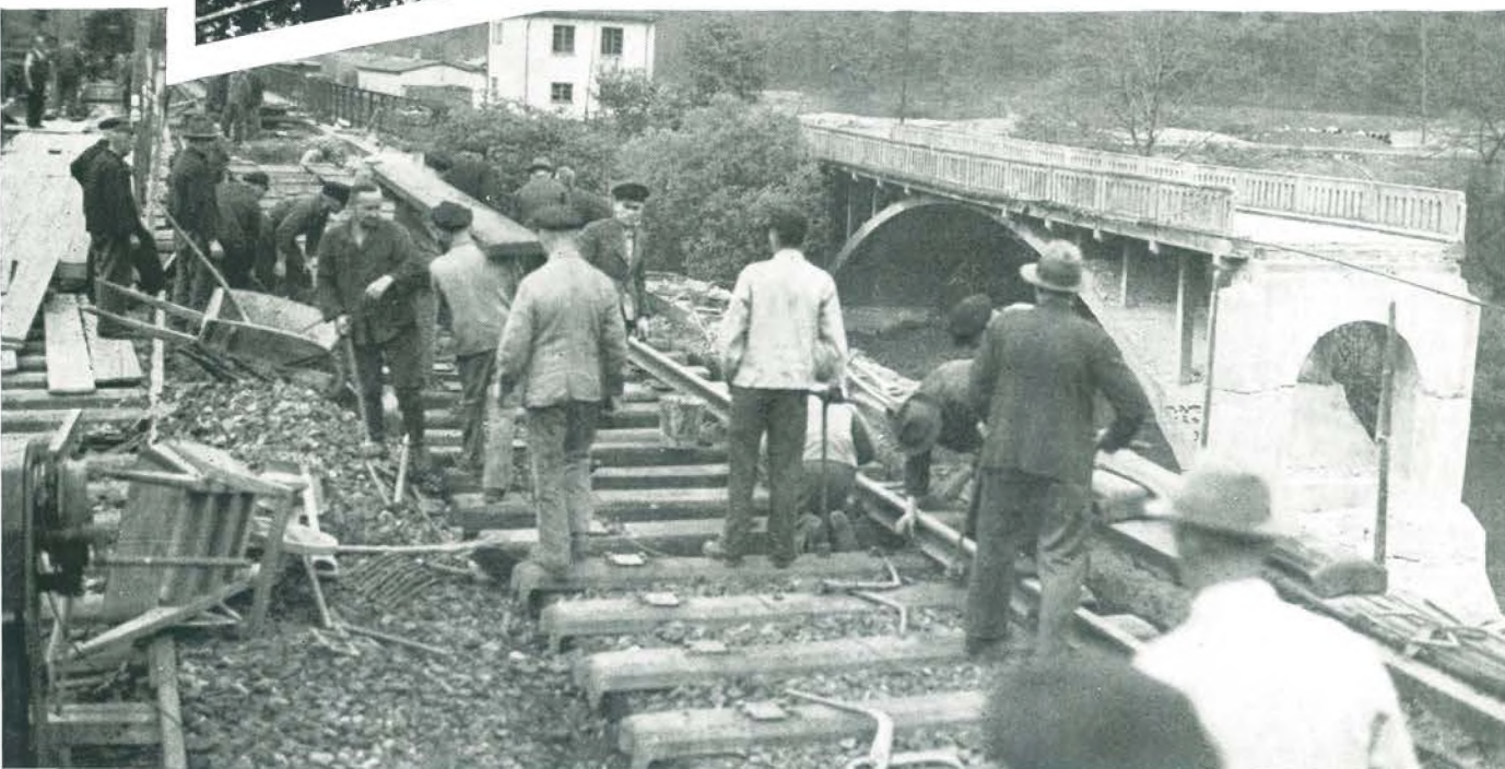
The remains of German munitions train which caught fire in tunnel are dragged out onto sidings to allow the passage to be cleared and repaired. Below German laborers lay rail on one of the very many rail bridges which had to be rebuilt to insure the carrying of material for the section reconstruction and rehabilitation of the area.
