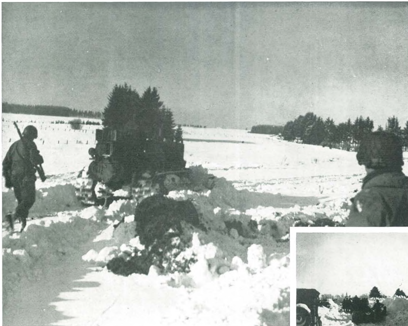
BULLDOZERS HAD THE JOB OF CLEARING THE SNOW SO THAT ROADS COULD BE IMPROVISED
