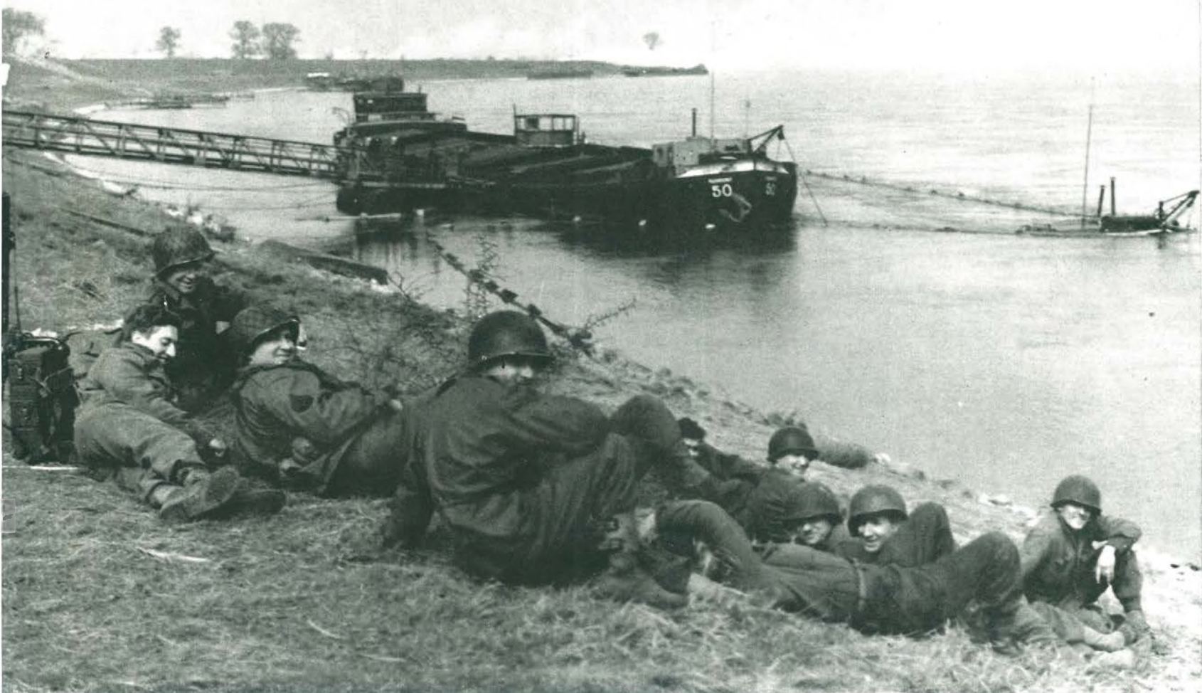
Smoke pots can be seen burning in the distance to cover the bridge. Upstream a boom is under construction which will prevent floating mines from damaging
