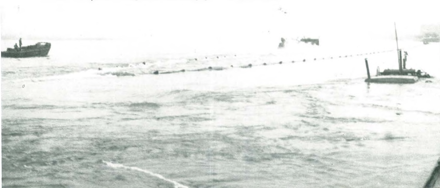
the span below (upper). Below is a shot of an LCM drawing a boom across the river to be securely anchored on opposite shore.
