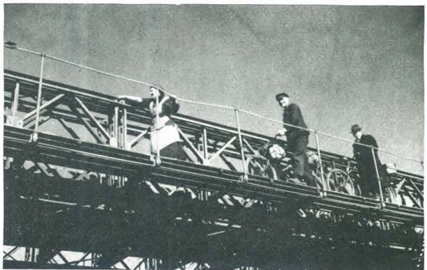
The new bridge was constructed next to the one which was blown out, and the operation was simplified since a great deal of the work was done on the deck of the old bridge below.
