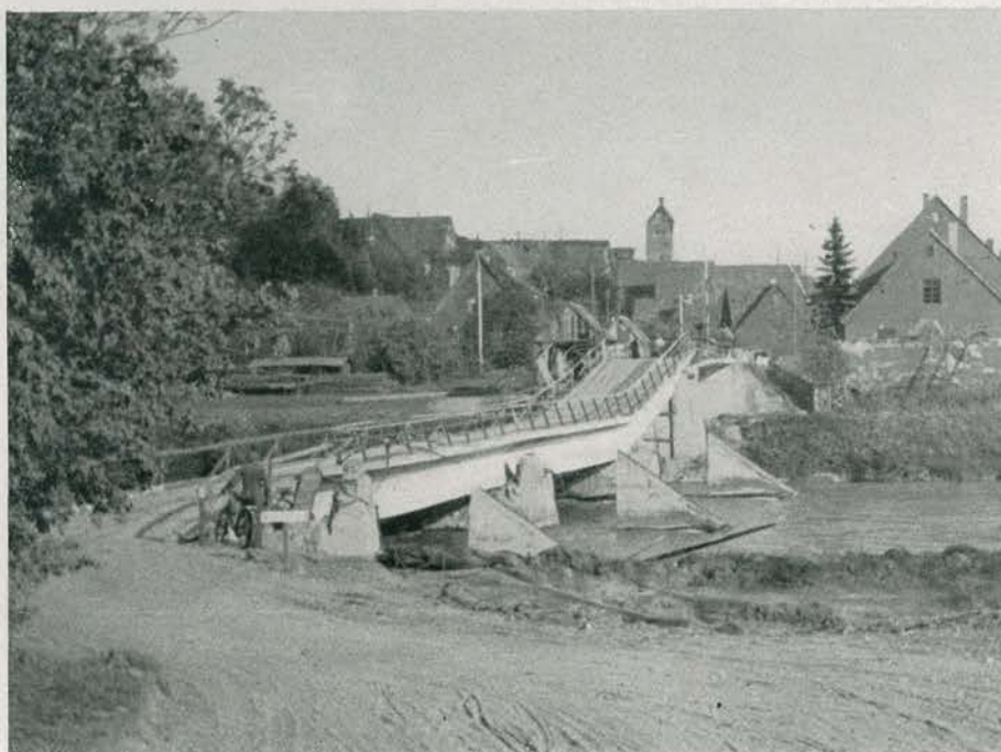
Another Danube bridge by 12th Armored Engineers. New structure is superimposed in the supports of the old bridge — south of Gundelfingen, Germany.
