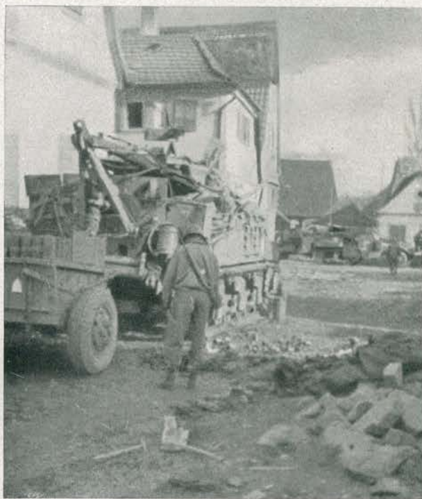
Motor maintenance worked day and night.
