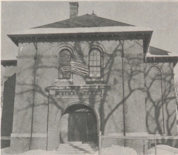
BANGOR'S NEW RECREATION CENTER
