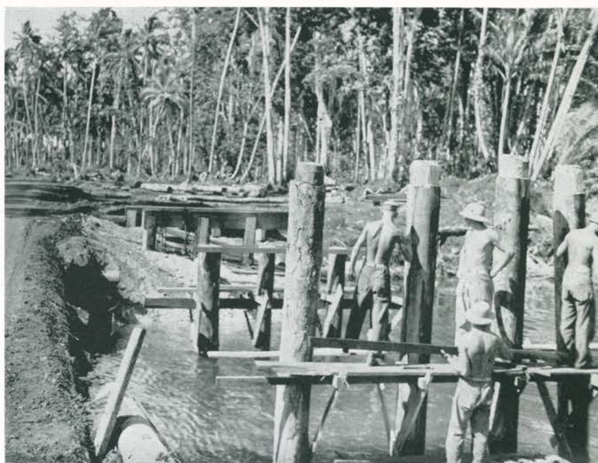
Reading from top to bottom: Improvised piledriver . . . hammer hits . . . they're down!
