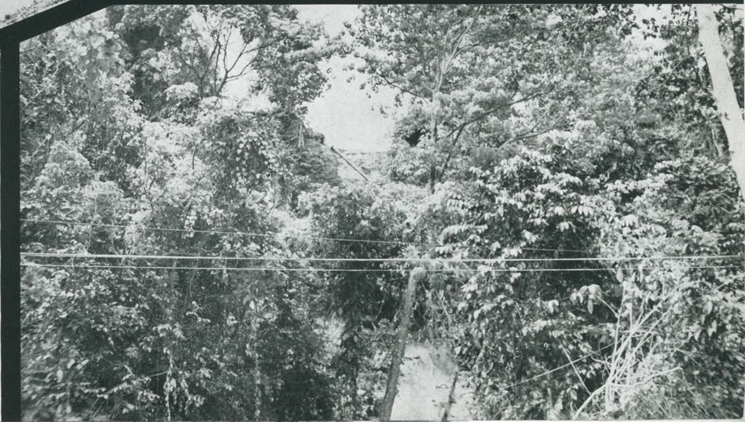
Pipeline Going Over Hill
