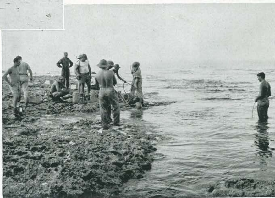
Setting Dynamite Under Water-Pilots' Pool
