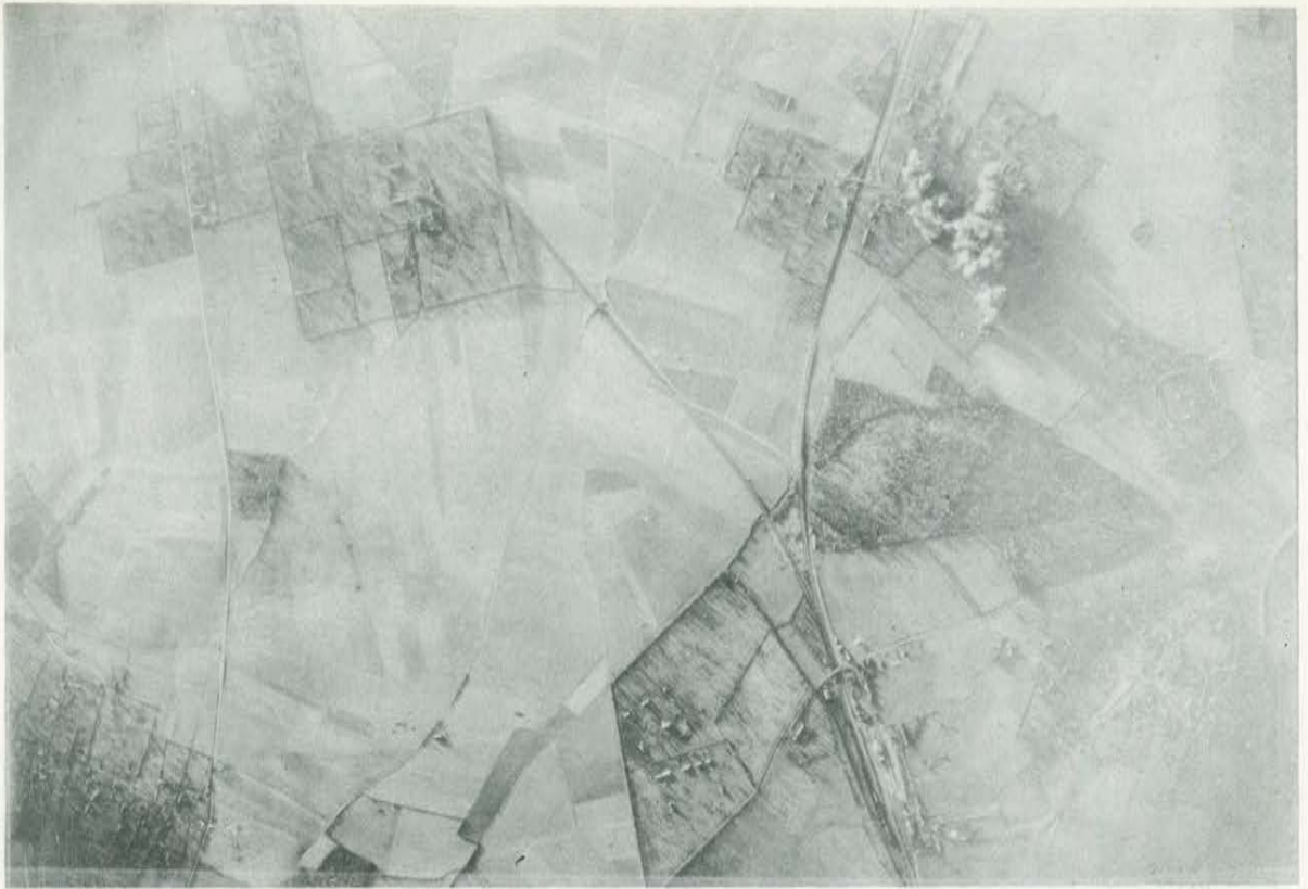
V-1 Launching Site, France, Jan. 14, 1944
