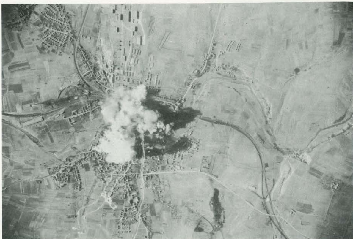
Crailsheim Railroad Yard, Germany, Feb. 23, 1945 After two concentrations of bombs had landed.
