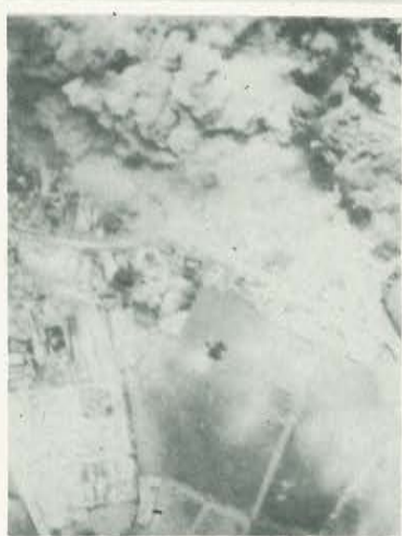
CARENTAN RAIL FACILITIES
