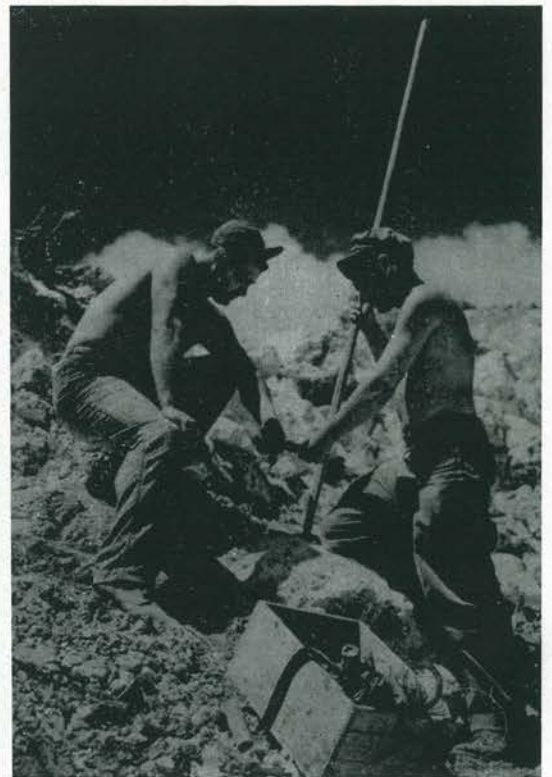
Harry Vorias and Al Failing tamp hole
