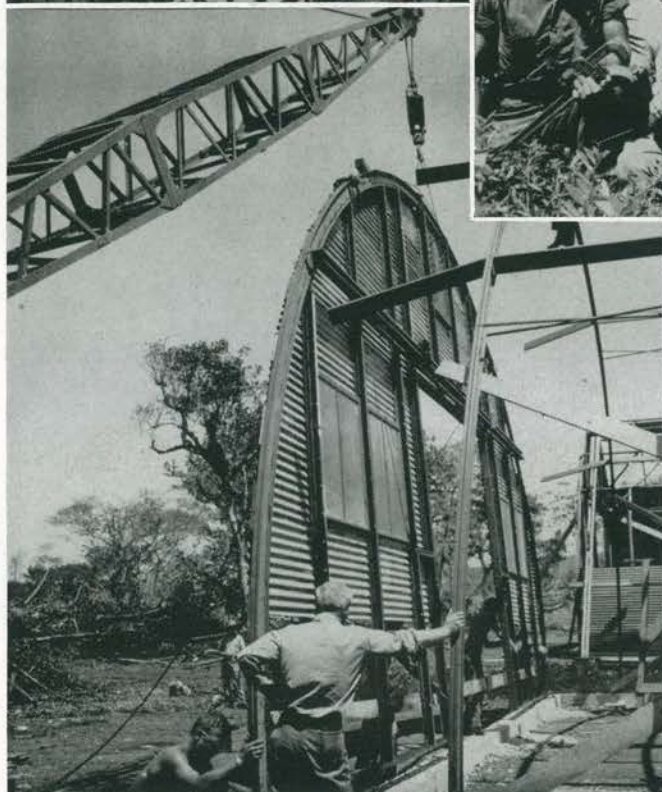
Quonset hut ribs go in a hurry Bulkhead of 40x100 warehouse set in place
