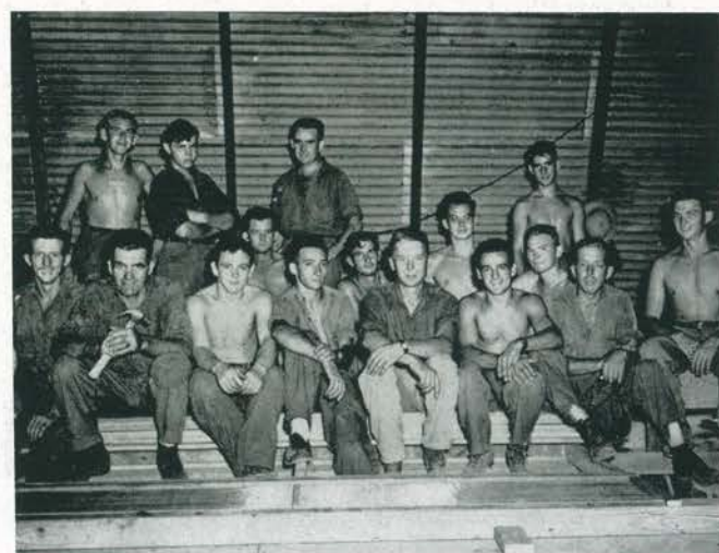
Prefabrication men readied material on time
