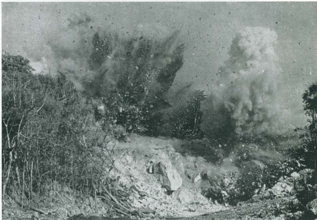
103rd powdermen at rock crusher brought forty per cent glycerine dynamite into use for facing
