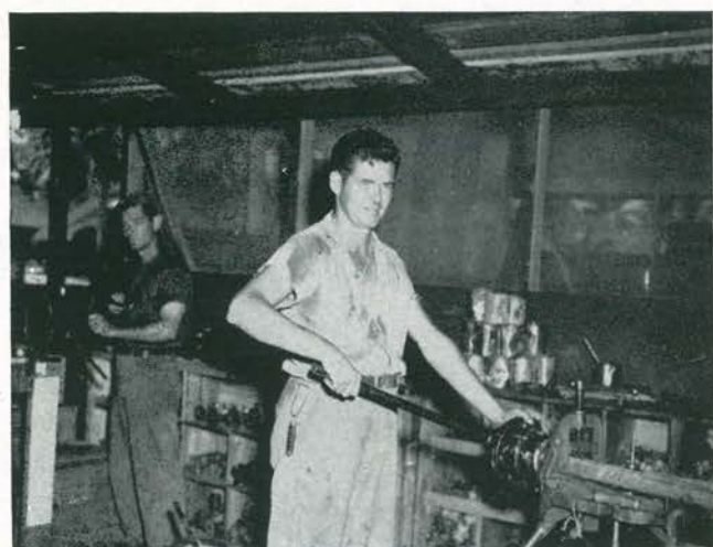
Area plumbing shop with SF1c's Long, Woodward
