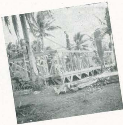
First work on camp sick-bay
