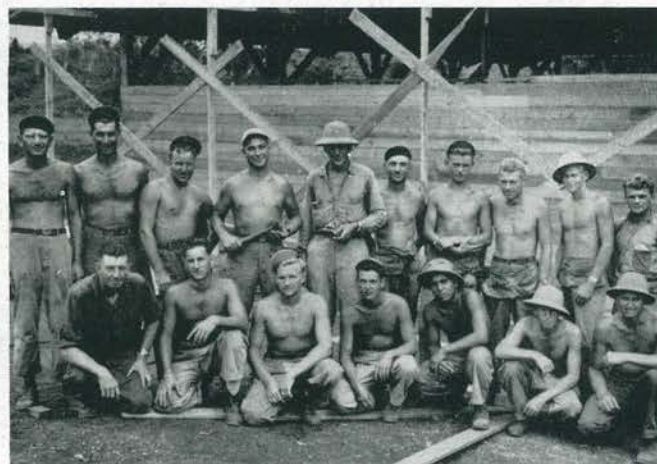
and Ludgate were Company A's erection gangs
