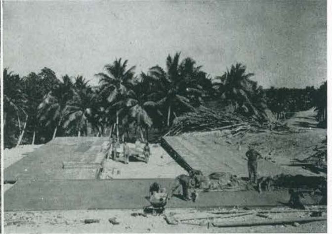
erected storage quonsets and built galleys for
