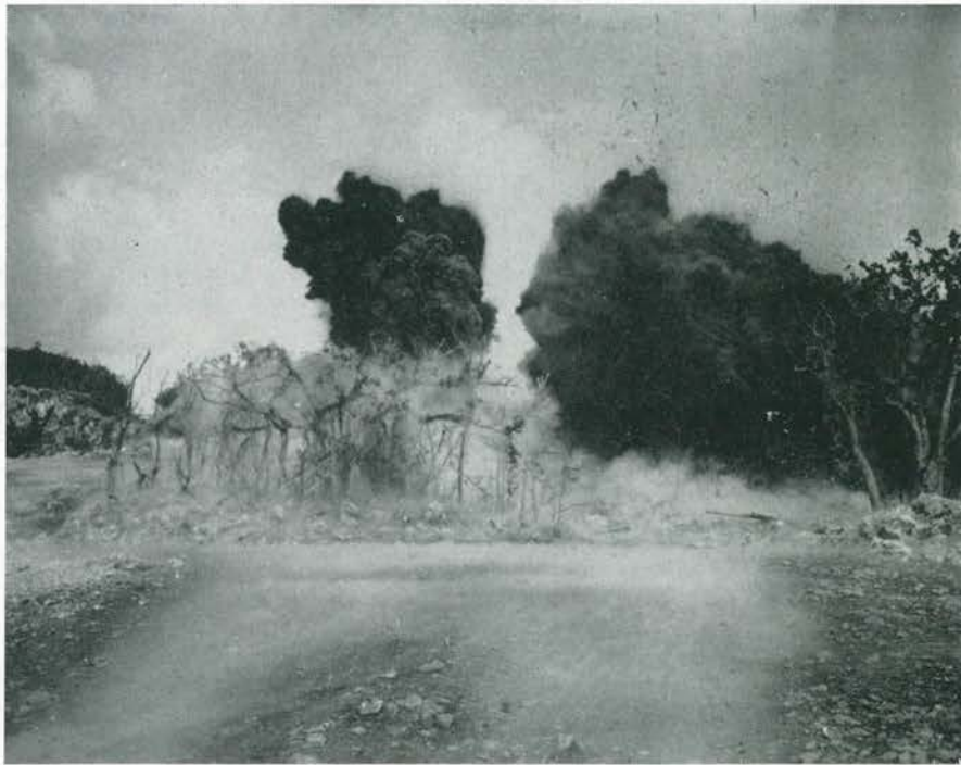
450 Bangalore tubes clear out jungle underbrush at rock crusher
