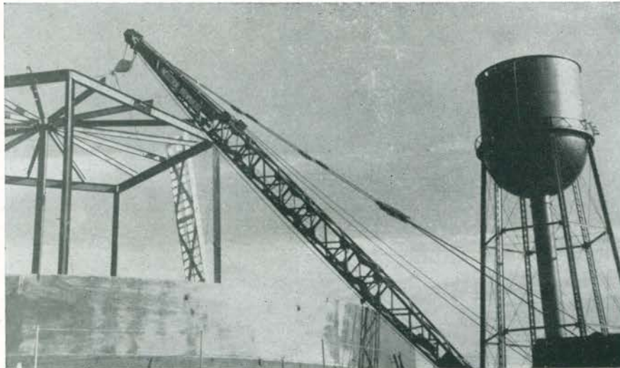
Welders work on 1,788,500 gallon tank across street from Kendall Hall
