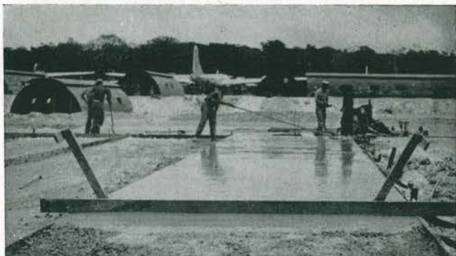
Slab-finishers at work on quonset office building
