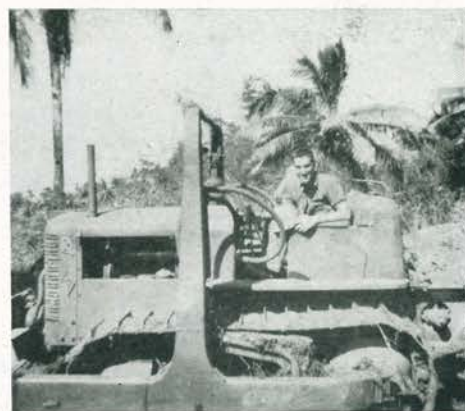
'Dozers cleared away the underbrush
