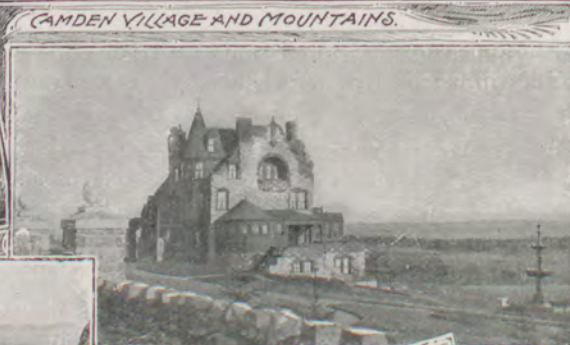
NORUMBEGA THE 18 STEARNS STONE WALL.
