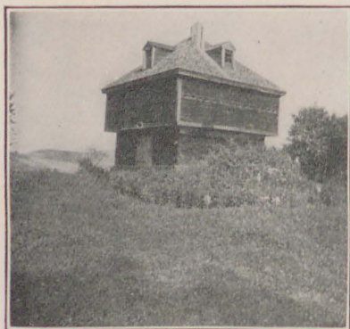
The Old Blockhouse at Fort Kent
