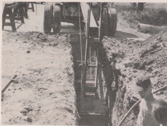
SEWER CREW AT WORK
