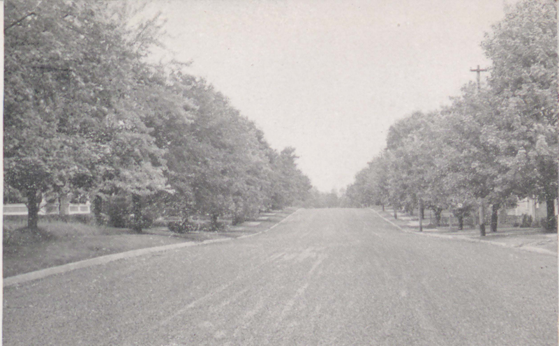
Royal Road rebuilt
