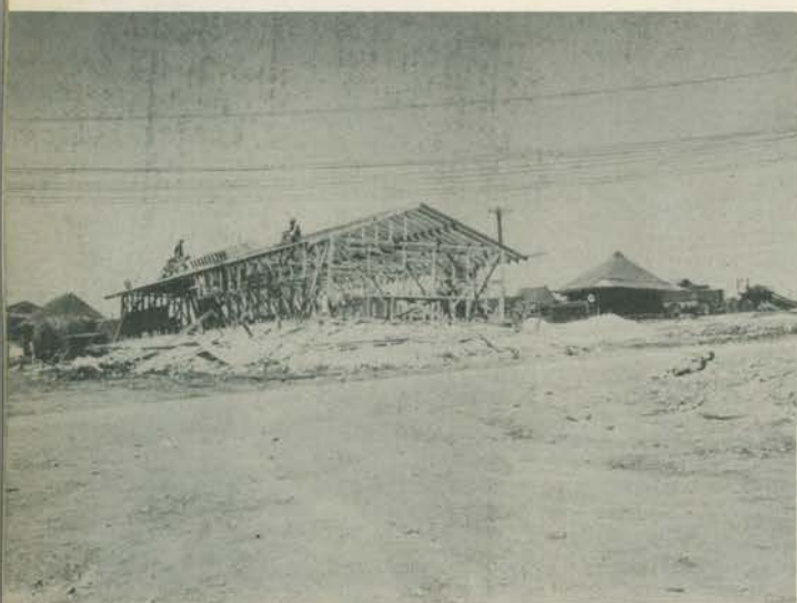
Mess hall construction—October 1944
