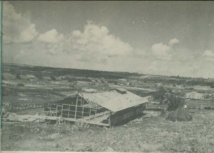
Mess hall (869th) construction—October 1944
