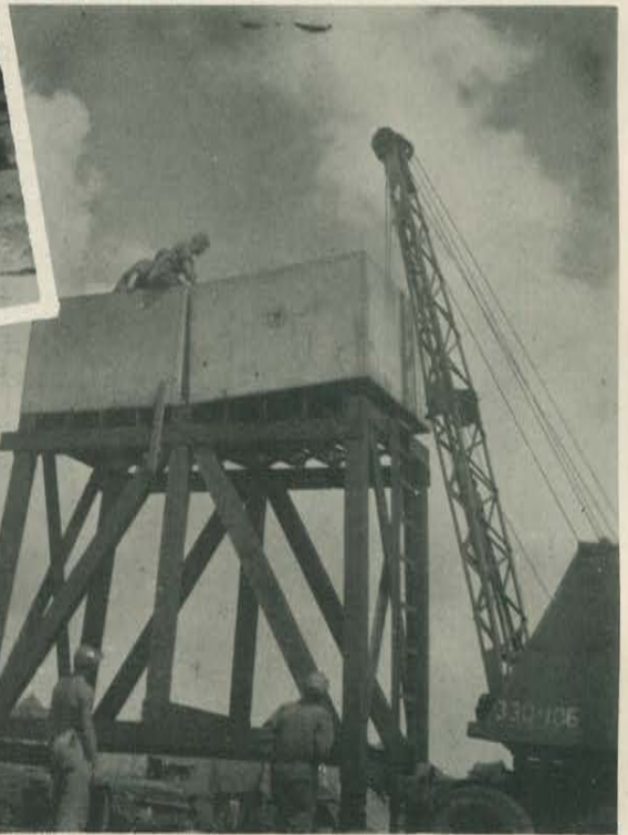
Erecting water tanks in October 44
