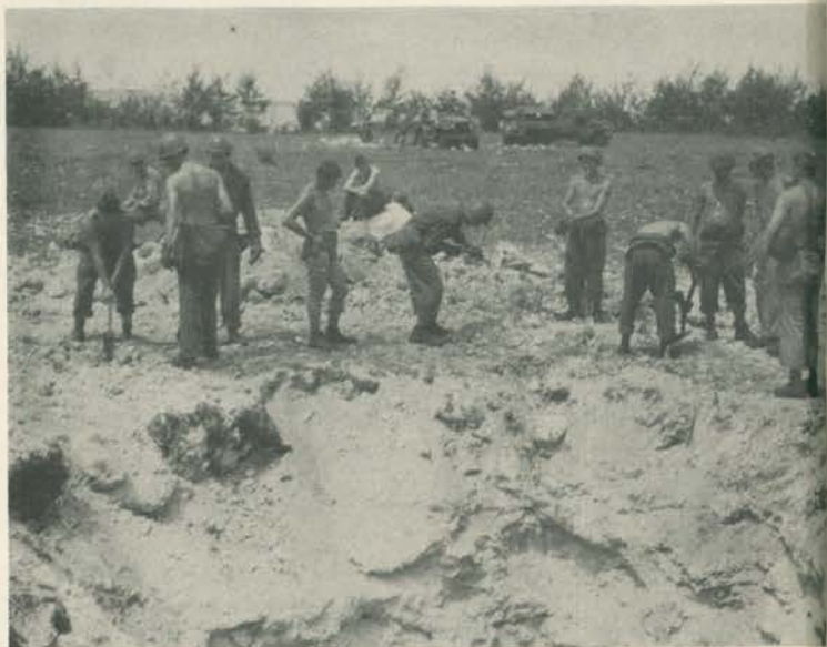
Beginning of latrine construction
