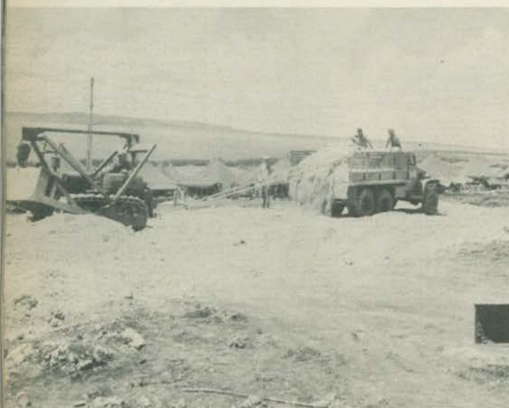
Road construction in September of 1944
