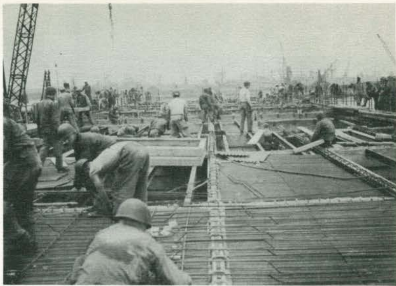
Working on the top deck
