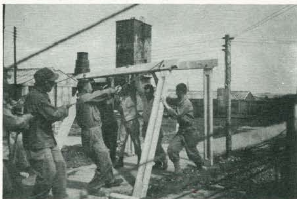
Work on a hospital
