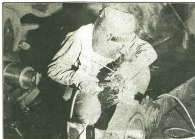
2. AND THE REPAIR
