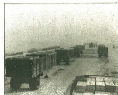
6. AT MARSHALLING YARD .....
