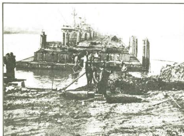
6. PIERS WERE BUILT
