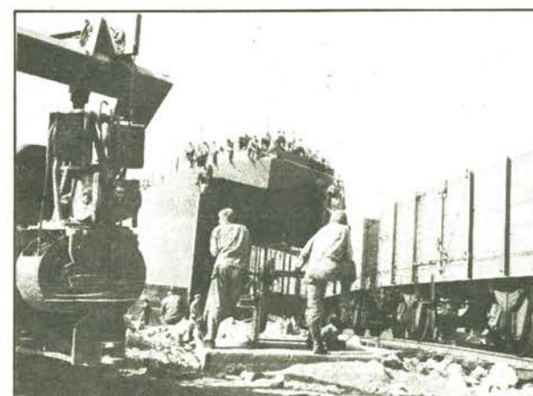
8. FERRYING HEAVY EQUIPMENT
