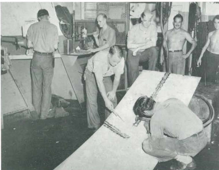
Shipfitters at work in shipfitter's shop.
