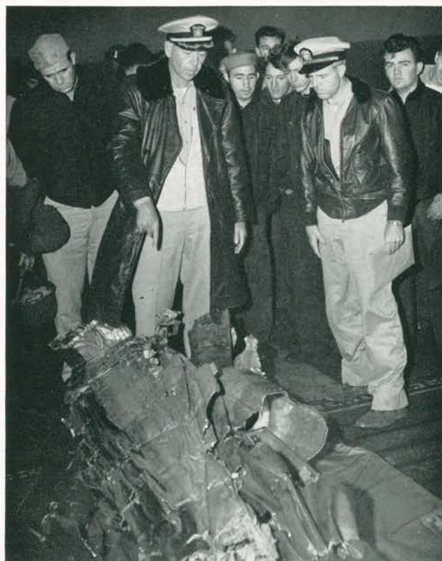
Captain and A.C.I. officer inspect wing section of Kamikaze left on our flight deck after hitting after part of island structure.
