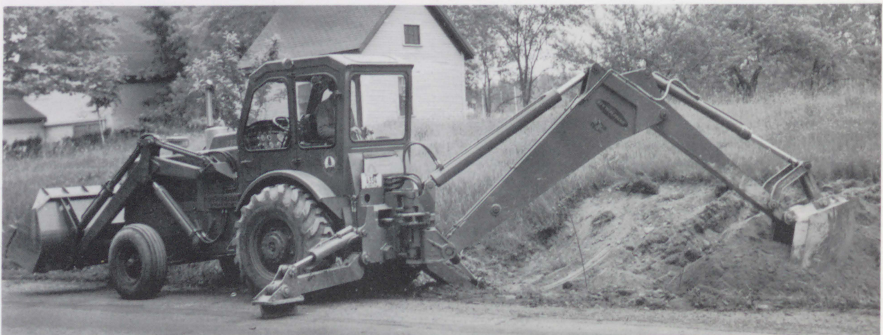
NEW BACKHOE IN OPERATION
