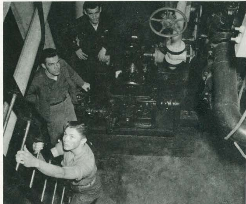
Fuel Oil Maintenance Crew and Equipment
