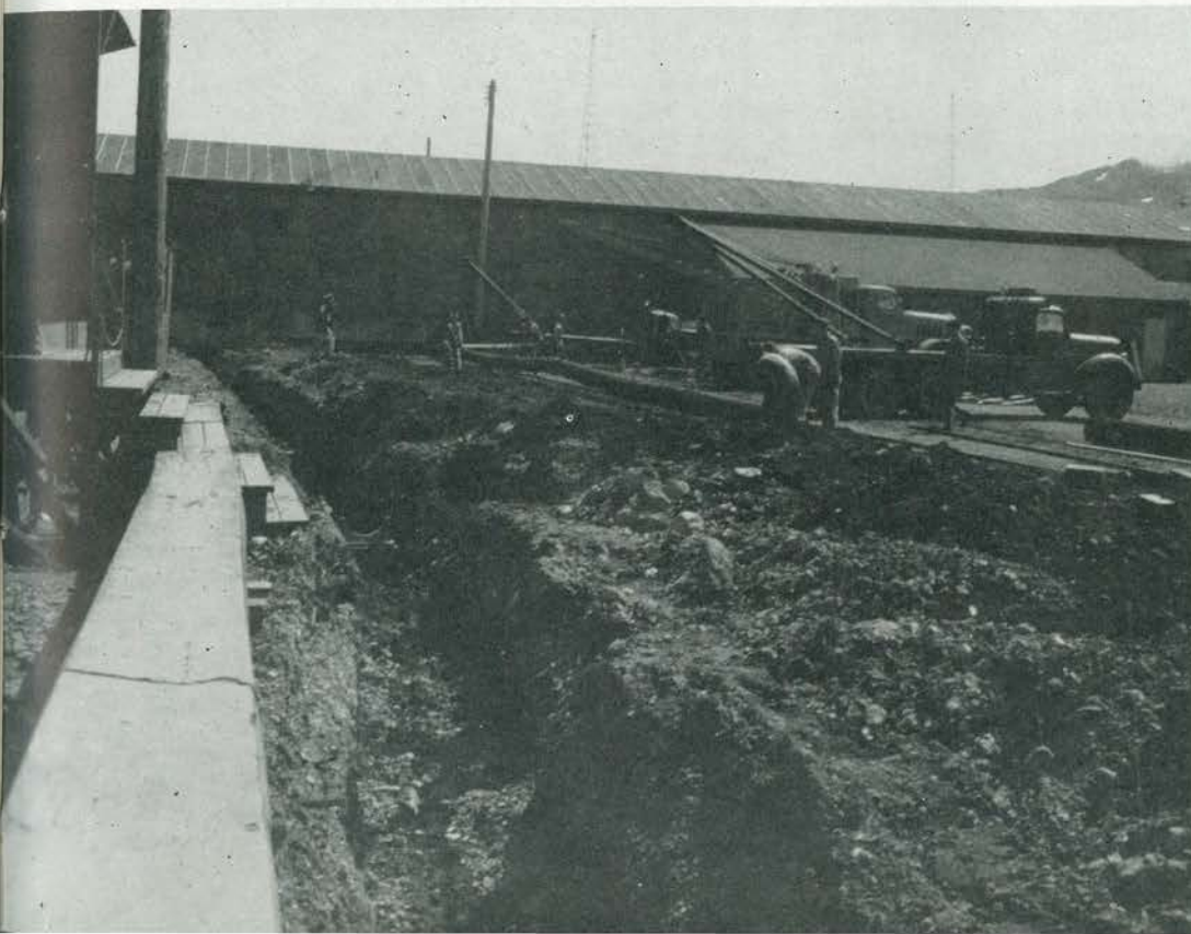
Placing Steam Line
