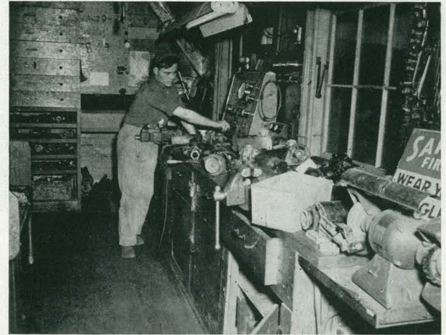
Repairman at Work in the Carburetor, Starter and Generator Section of the P.W. Garage
