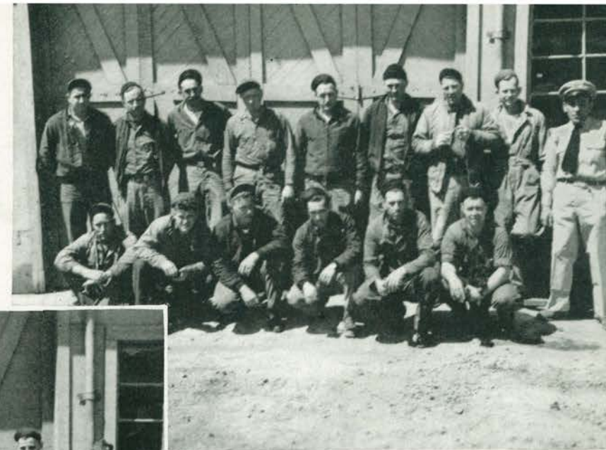
Road Maintenance Crew
