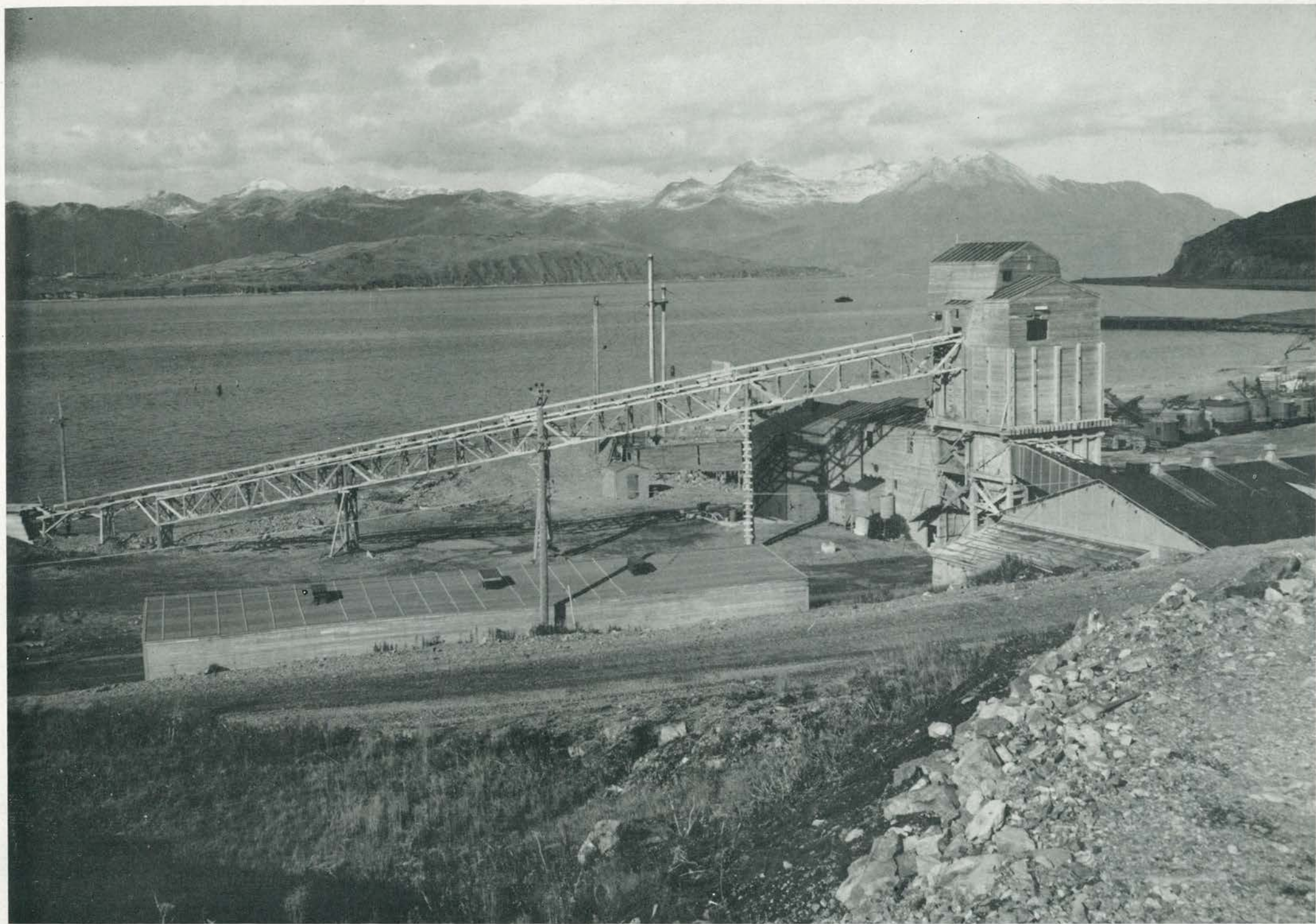
AGGREGATE PLANT WITH HOG ISLAND IN BACKGROUND
