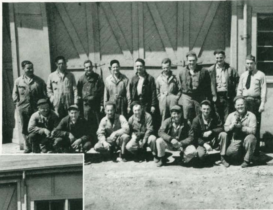
Road Maintenance of CB Shops Crew
