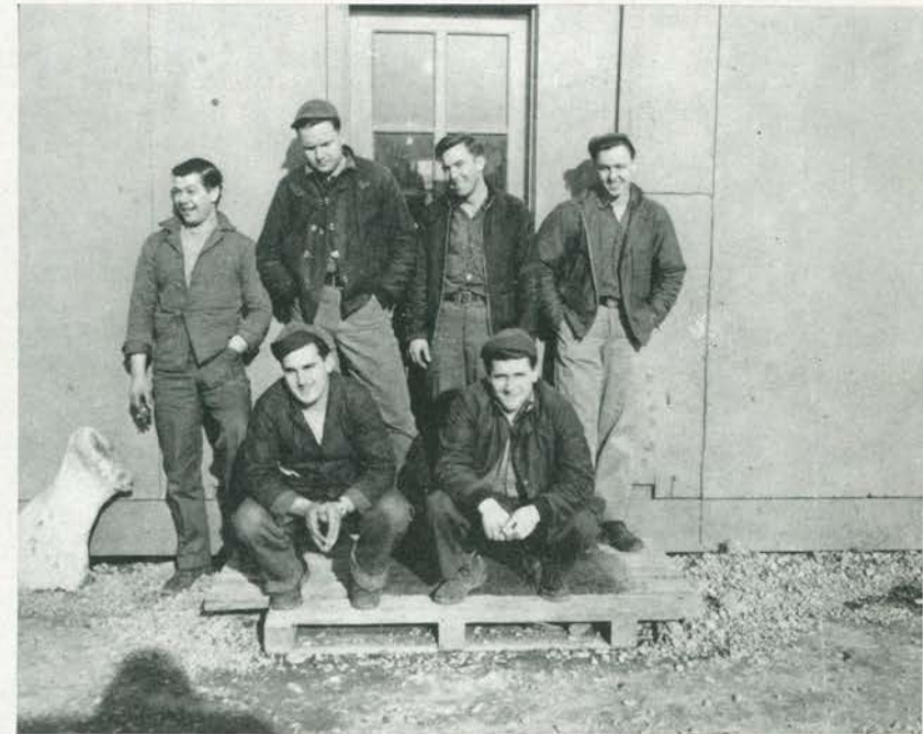
Fuel Oil Distribution Crew
