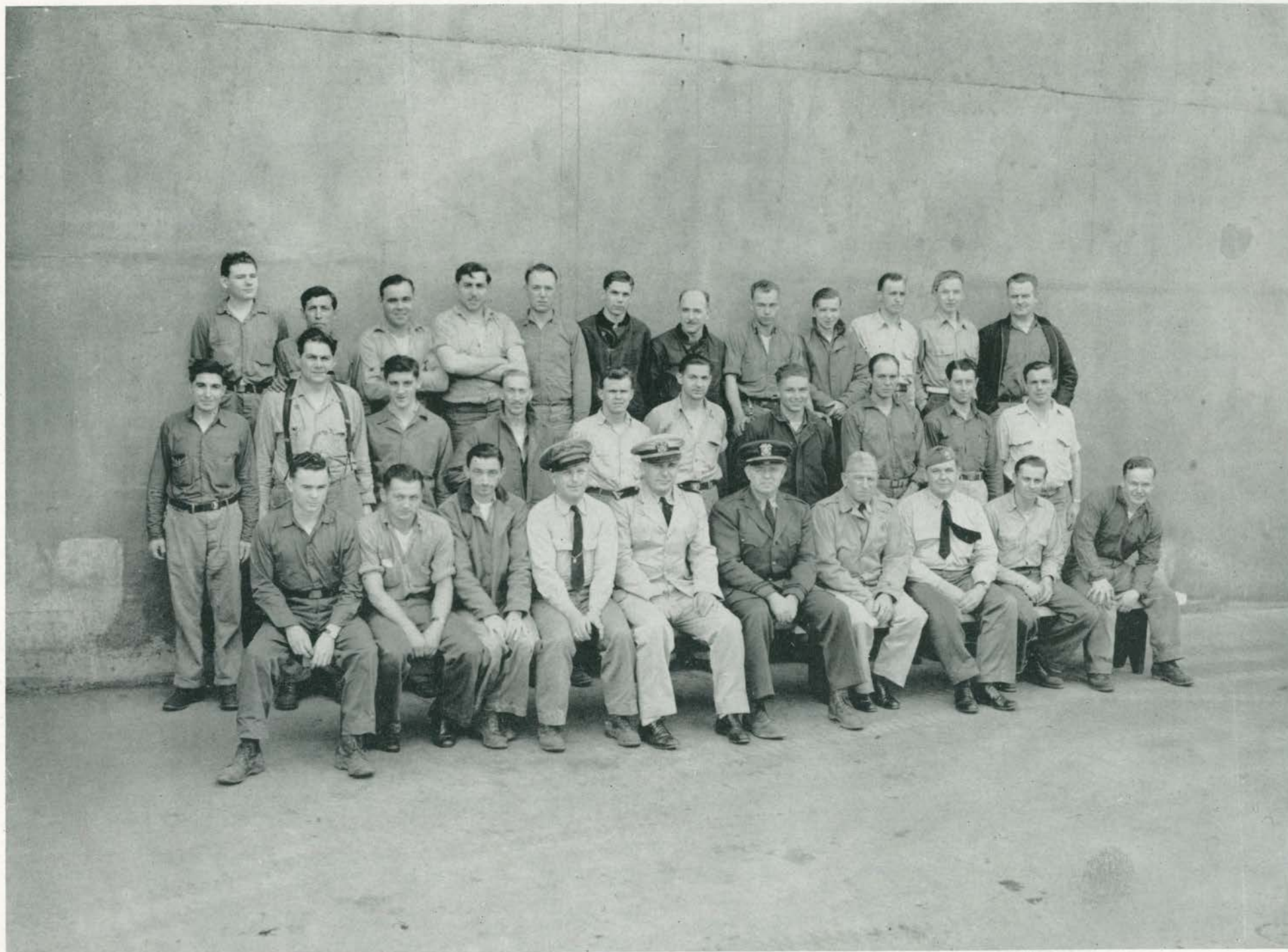
NOB POWER PLANT CREW
