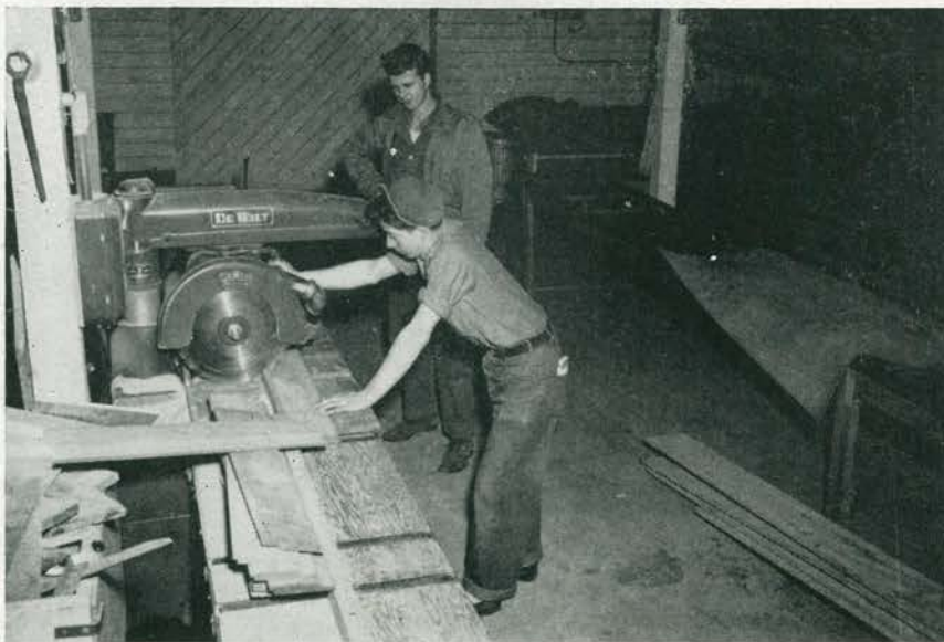
Interior of Carpenter Shop
