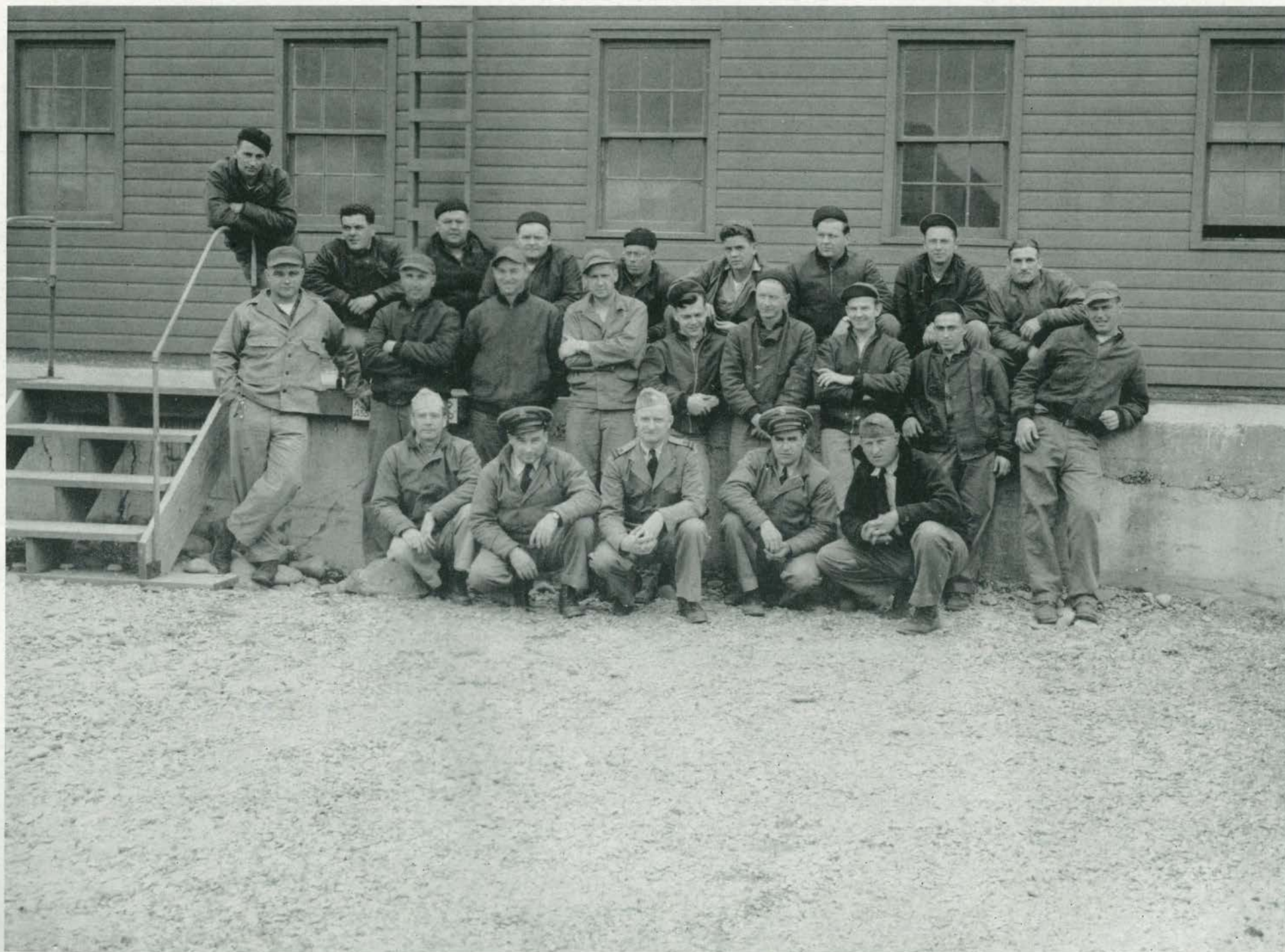
ELECTRICAL UTILITIES AND TELEPHONE CREW
