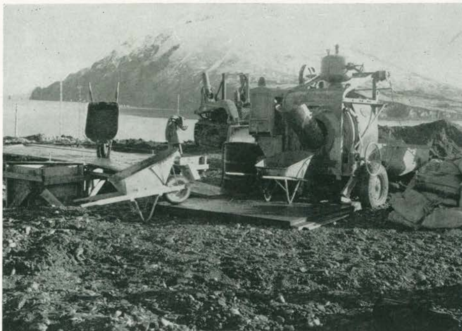
Pouring Foundation for East Tower
