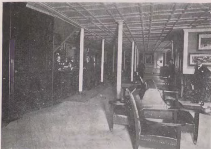
Office, Bangor House, Bangor, Maine
