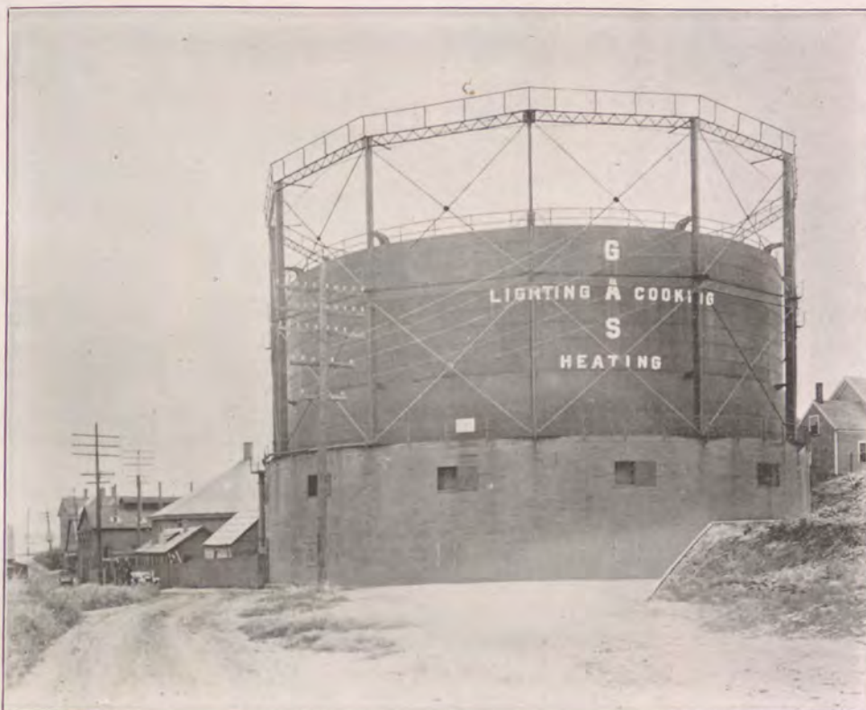
Bangor Gas Light Company's Plant
