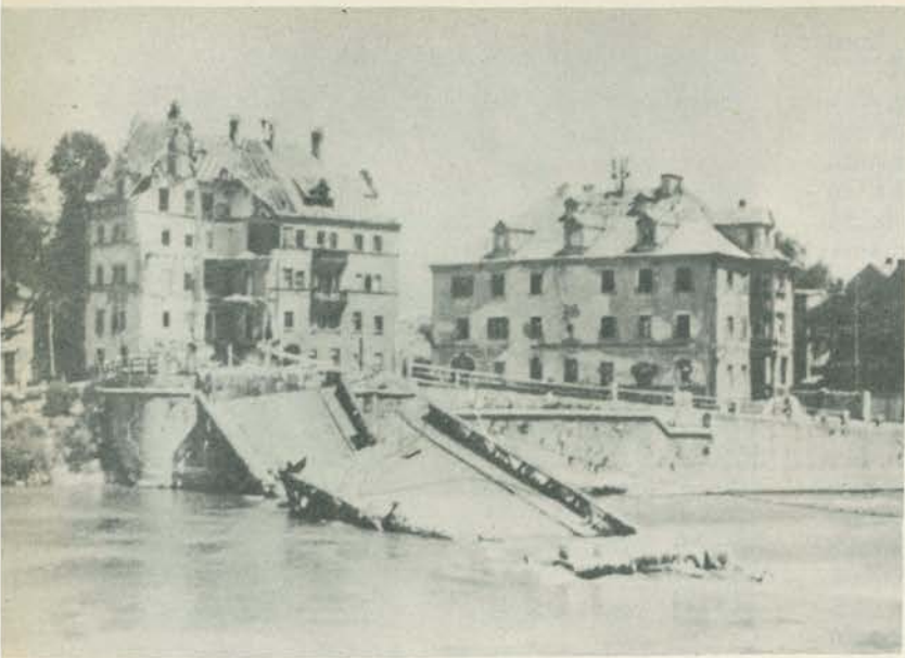
Bridges destroyed by the Germans at Regensburg
