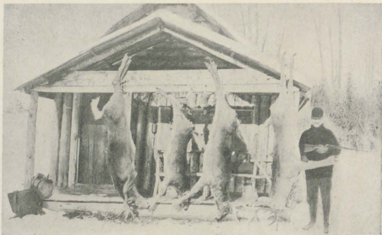
At Katahdin Iron Works
