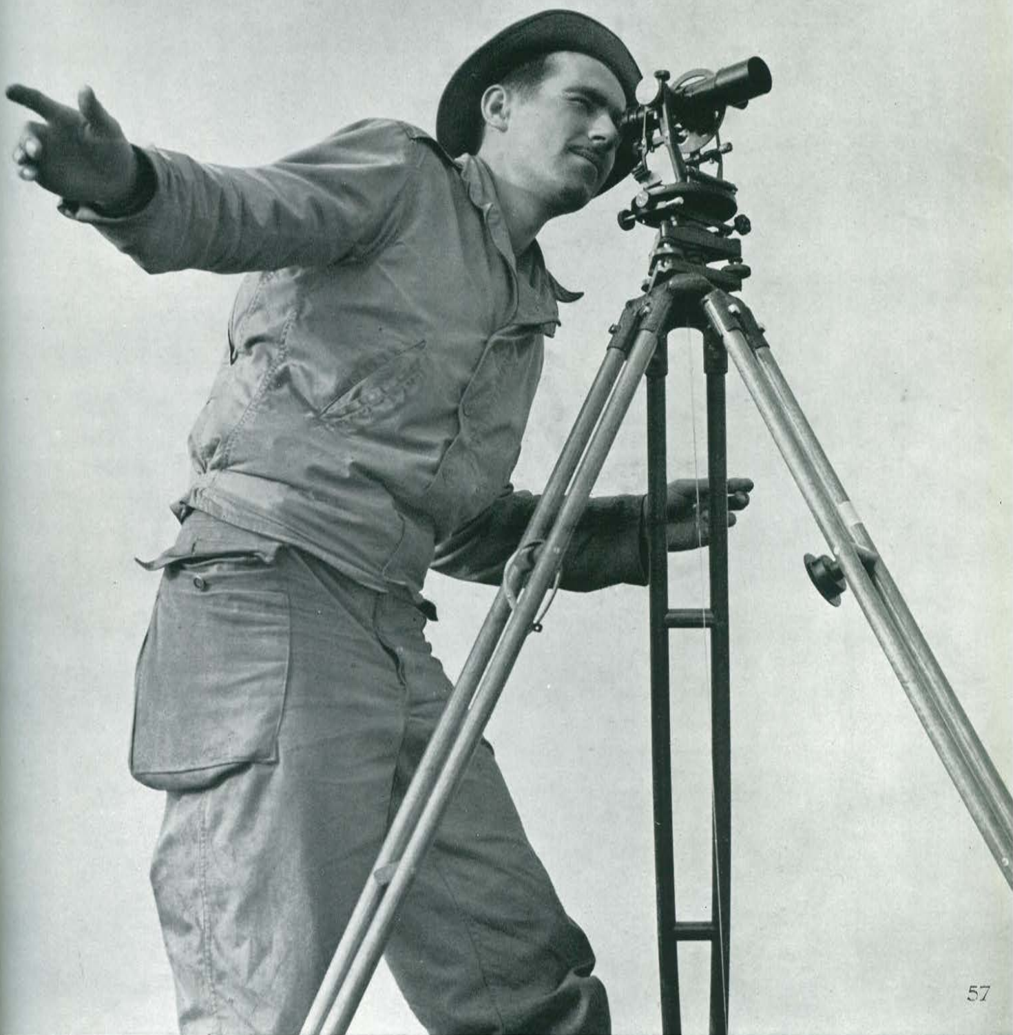
John Trask sighting the centerline for a new runway.
