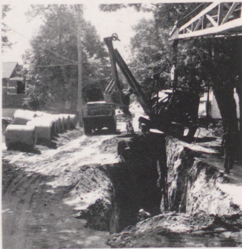
Fourteenth Street Sewer Rebuilt
