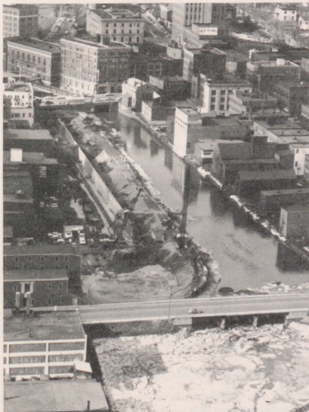
Kenduskeag Parking Project takes shape
