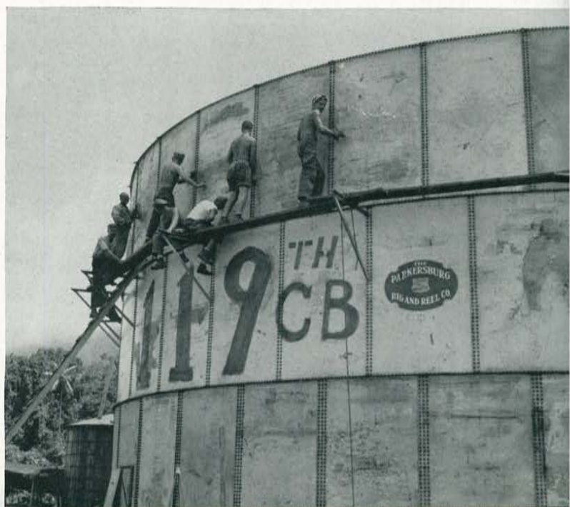
A final check on the bolts.
