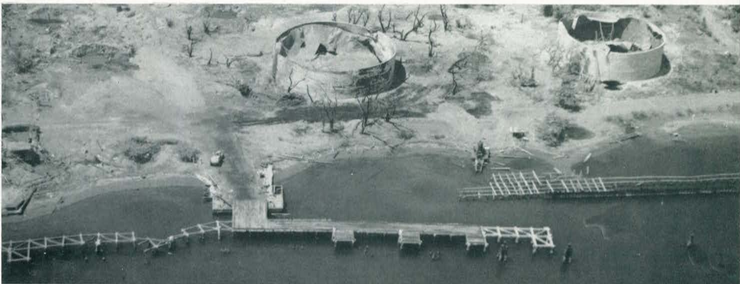
Wrecked docks and fuel tanks at Cavite.
