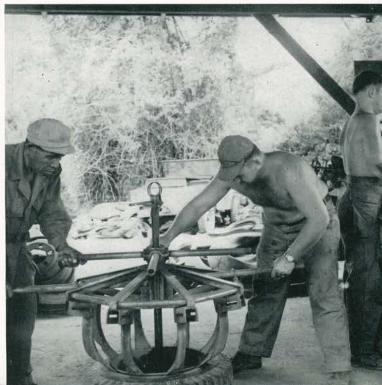
Filipino mechanic helps 119th USNCB tire men fix flat.
