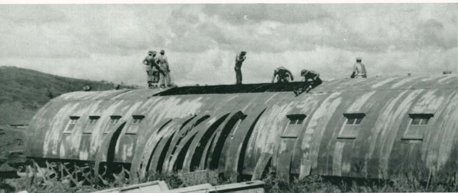
Another hut will soon be completed.
