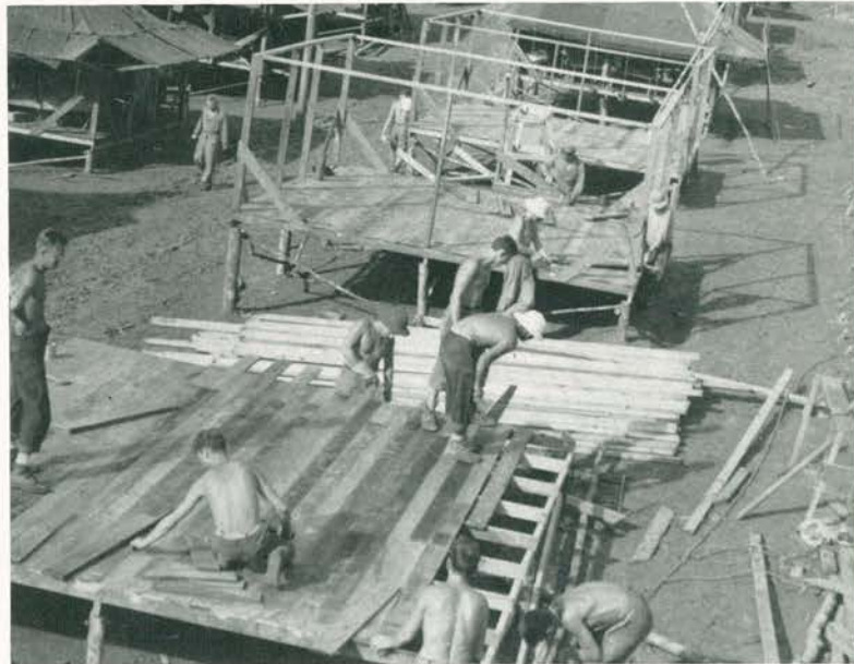
Building the enlisted men's quarters.
